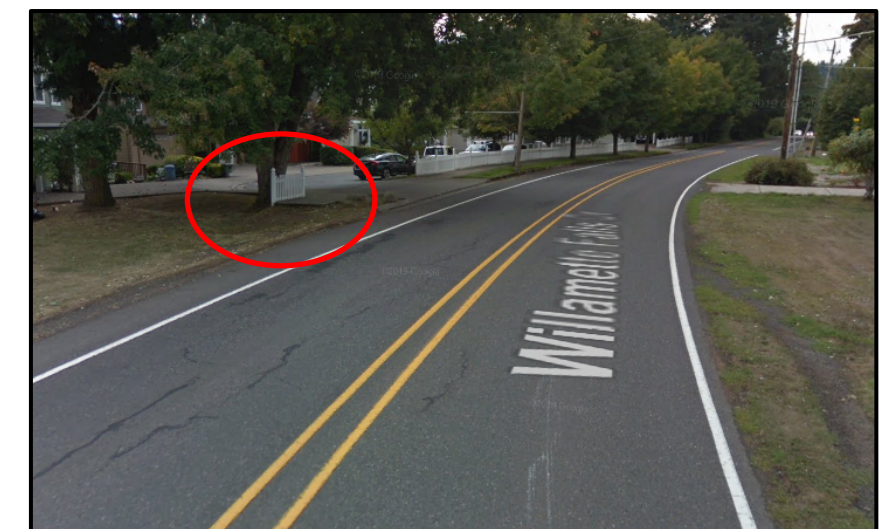
Sidewalk ends short of connection to downtown
