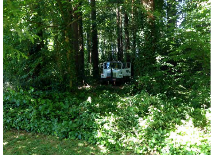
Photograph 2: Drill rig at boring B-3.
