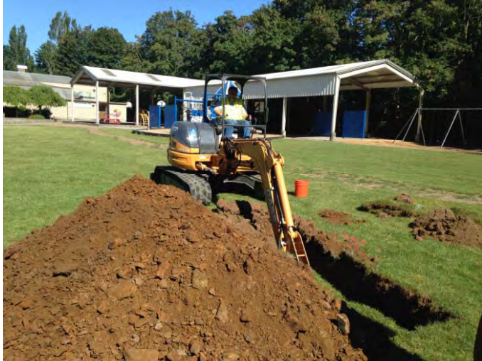
Photograph 1: Excavation of test pit TP-1 in progress.
