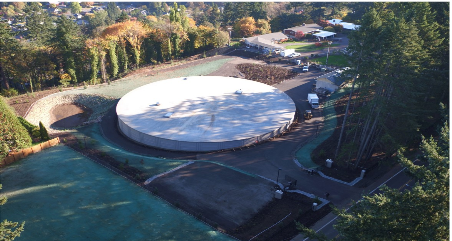
West Linn's Bolton Reservoir before and after pictures. 100 year old 2.5 MG tank pictured above and New 4.0 MG tank pictured below
