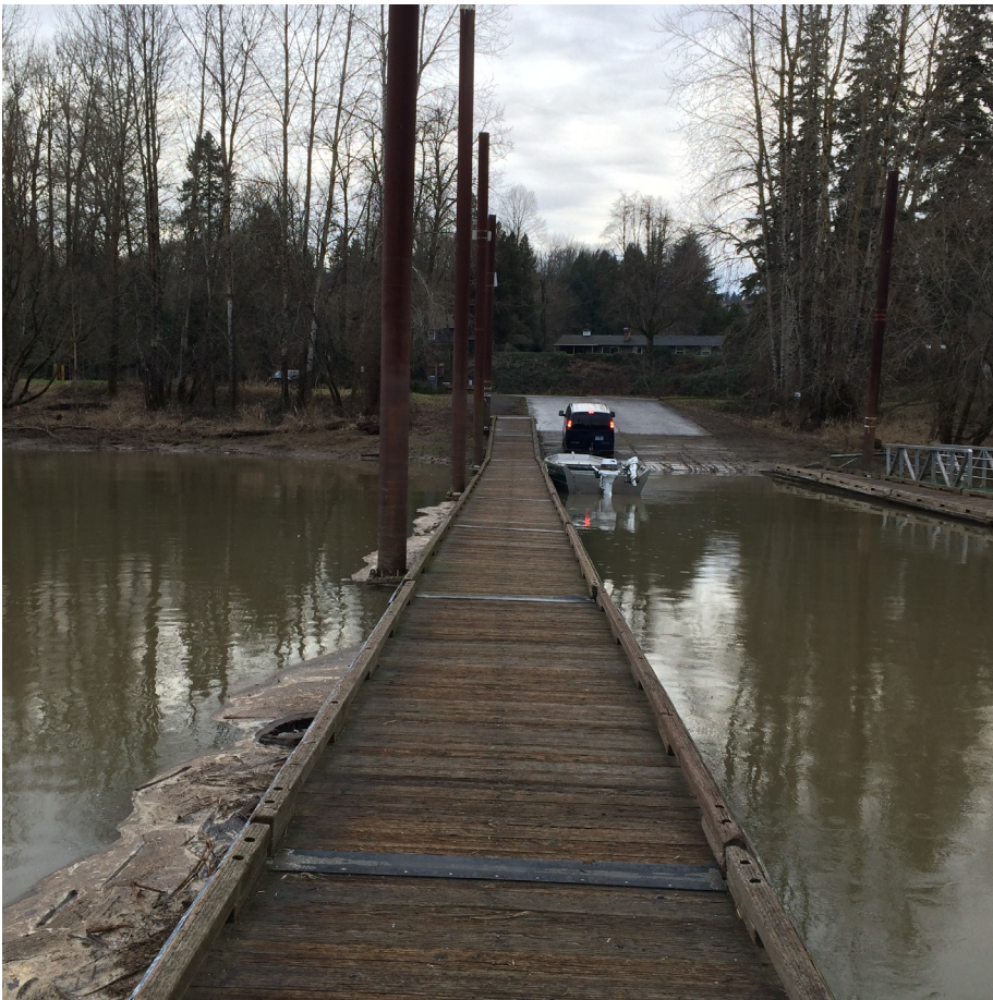
Photograph 8: Existing boat docks and ramp
