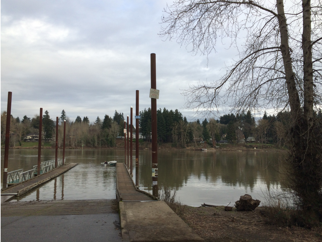
Photograph 7: Existing boat docks and ramp
