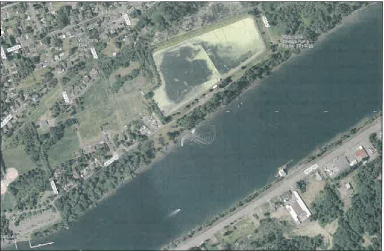
Image 1 Site Aerial View
