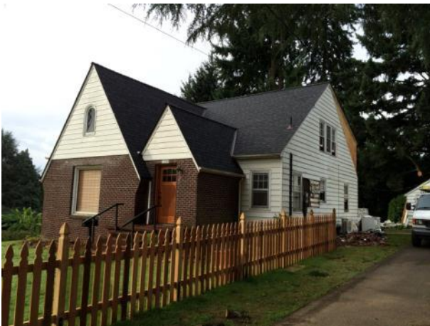
October 2013 – Front and side (north) elevation
