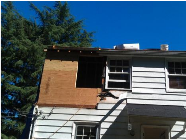
Rear elevation – September 2013
