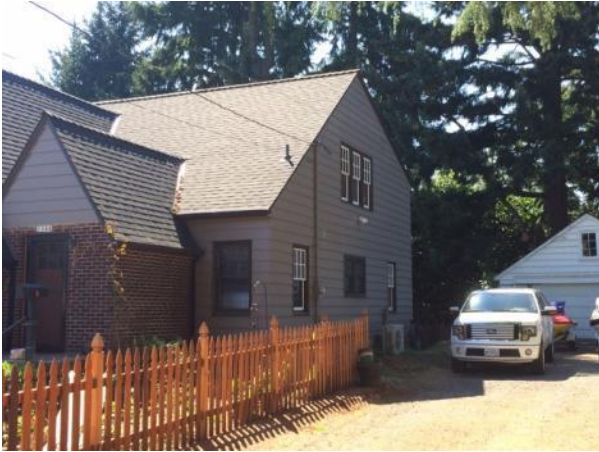
Side (north) Elevation – August 2014
