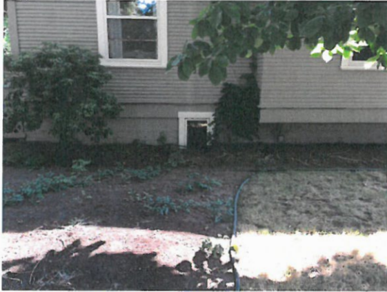
Existing basement window and well
