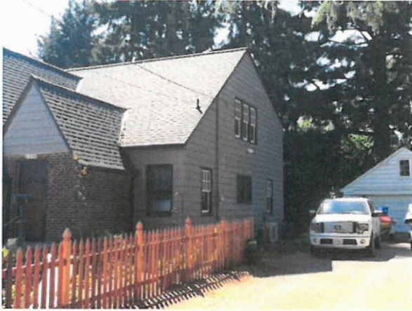
October 2013 – Front and side (north) elevation
