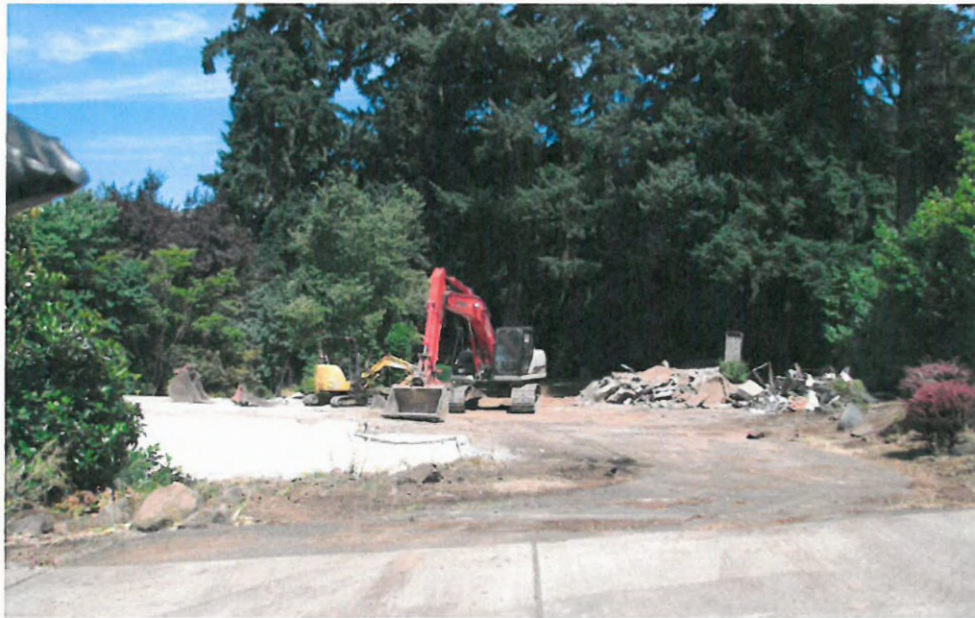
View from Remington Drive after house and garage demolished.
