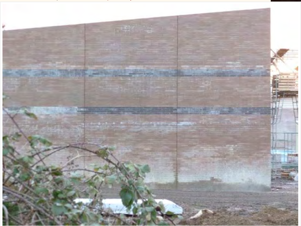
The efflorescence on the play structure detracts from the neighborhood. The notion of 'white elephant' comes to mind.
