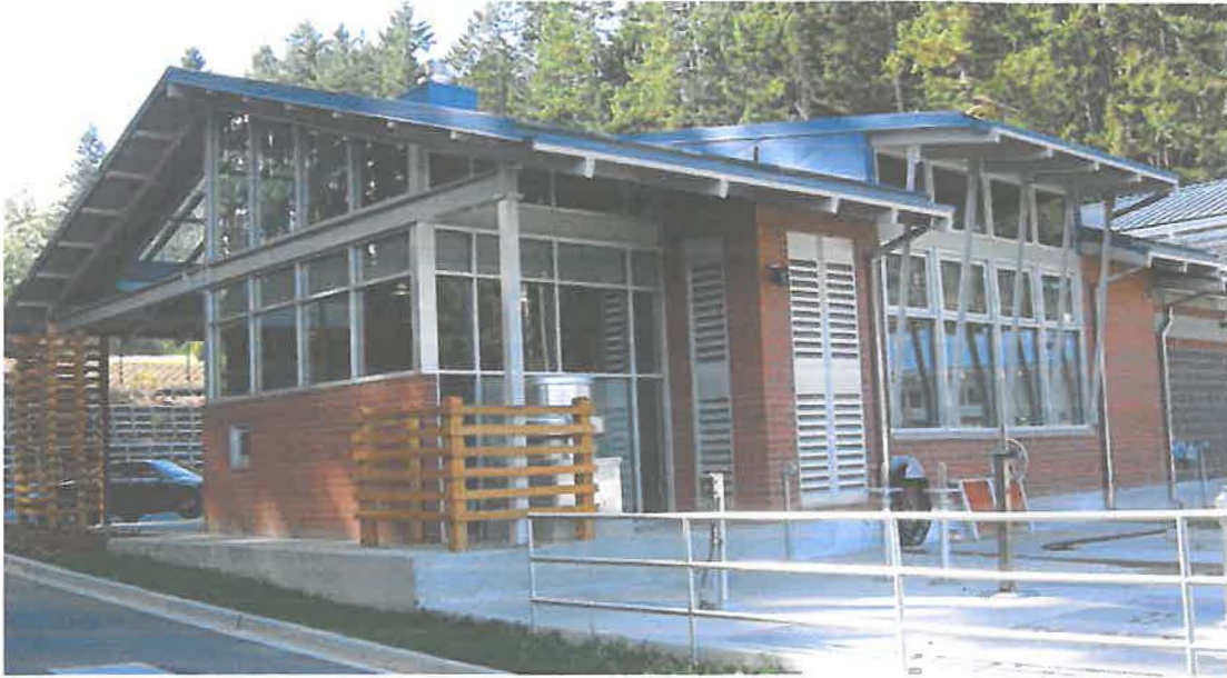
Figure 2 - Lacy-Olympia-Thurston-Tumwater Wastewater Treatment Facility by Michael Willis Architects
