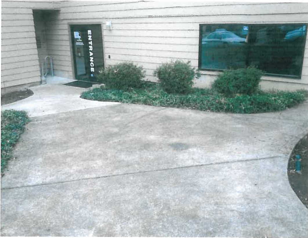
Area on 8 th Avenue side of building.
