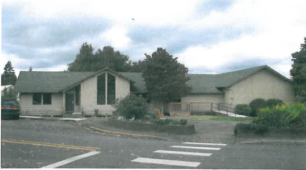
Front façade of building, set at angle facing 10 th Street/Willamette Falls Drive intersection. Although this is the visual front of the building, the site has an 8 th Avenue address. 8 th Avenue is north of the site, parallel to Willamette Falls Drive.
