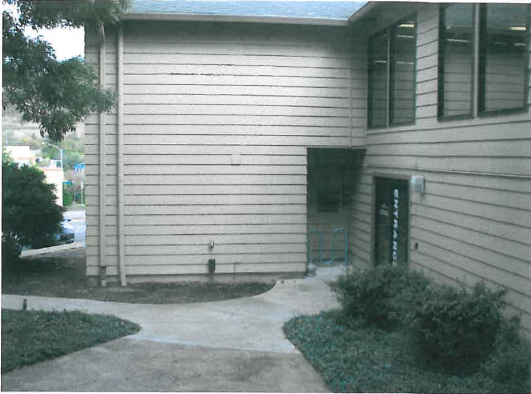
Existing covered bicycle parking in nook along rear façade of building.
