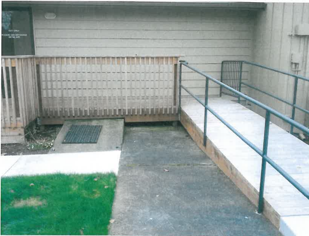
Area on Willamette Falls Drive side of building.
