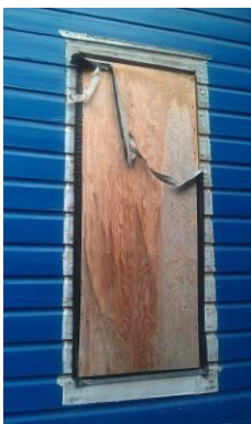
Existing side elevation window (2012)
