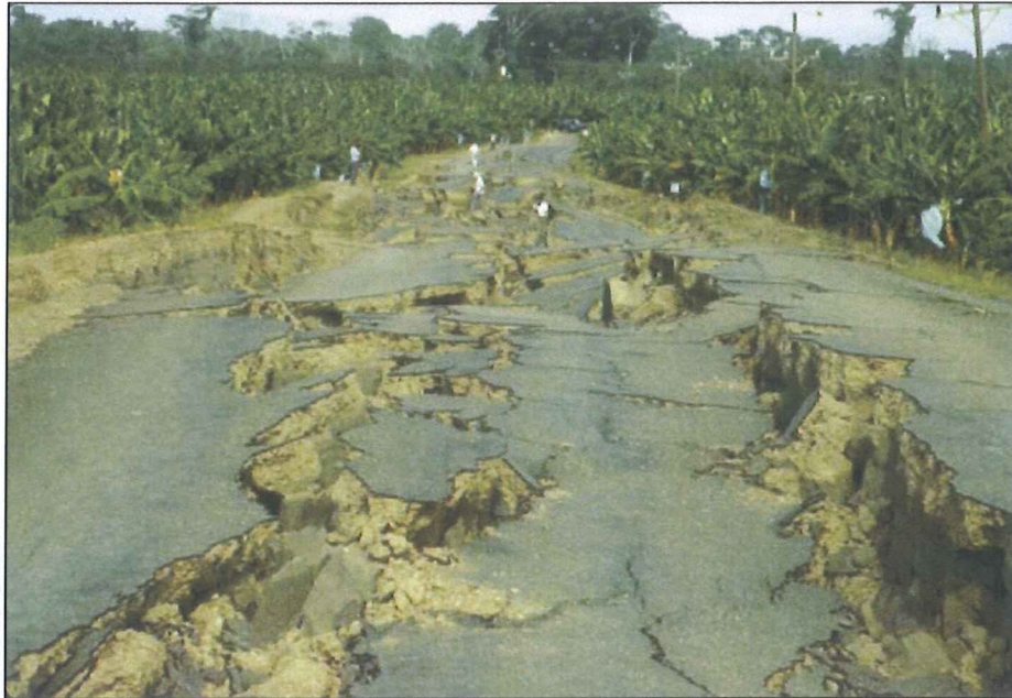
Permanent ground deformation, as occurred in the 1991 Limon, Costa Rica, earthquake, results from lateral spreading.
