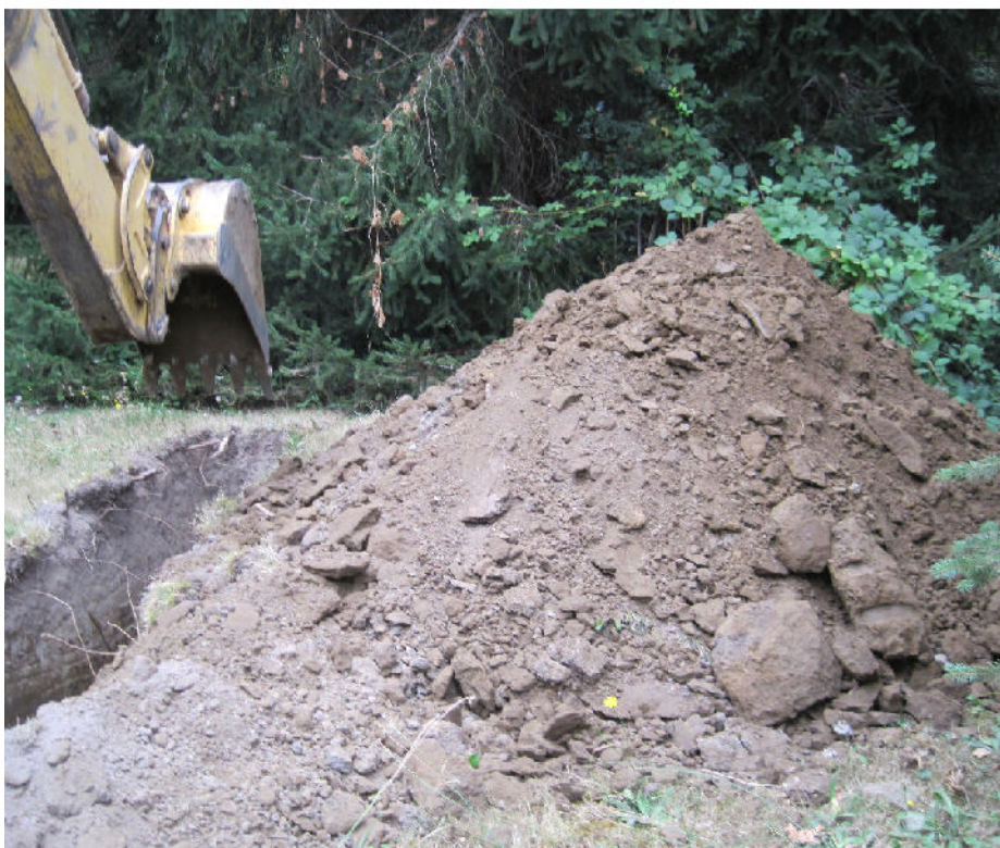
Photograph 4: Test pit TP-2 excavated material
