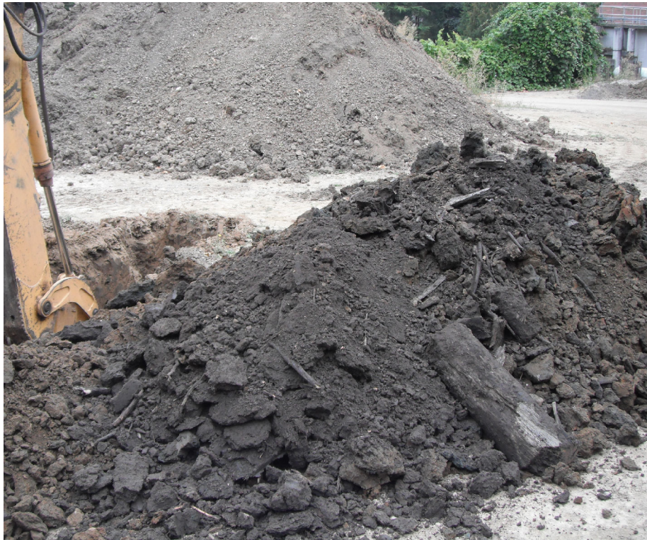
Photograph 2: Test pit TP-1 excavated material
