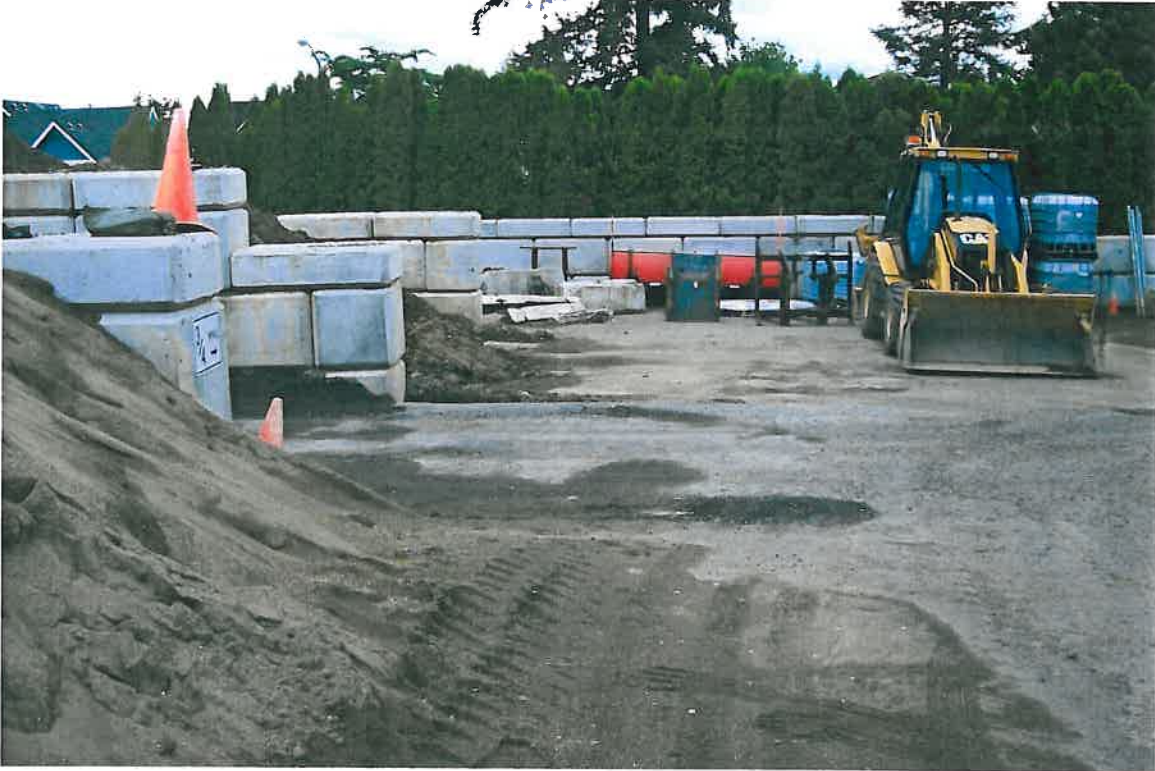
Materials Storage – Looking East
