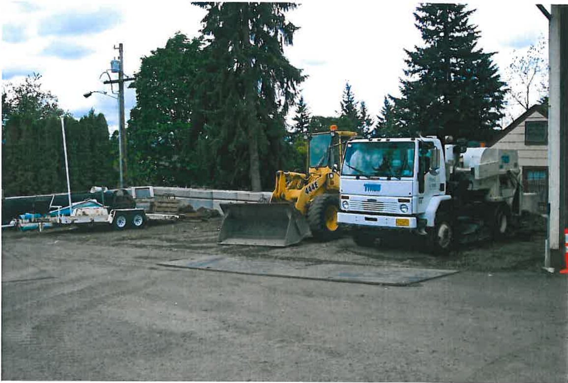
Covered Parking Building Site – Looking Southeast
