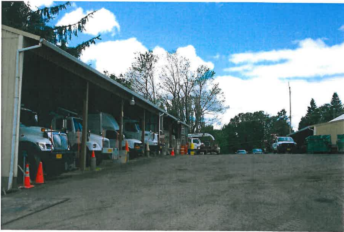
Equipment Parking Sheds Adjacent to Proposed Building – Looking West
