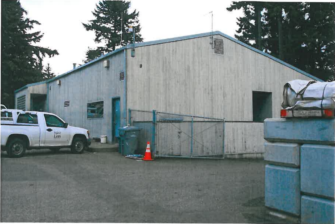
Administration Building – Looking Northeast
