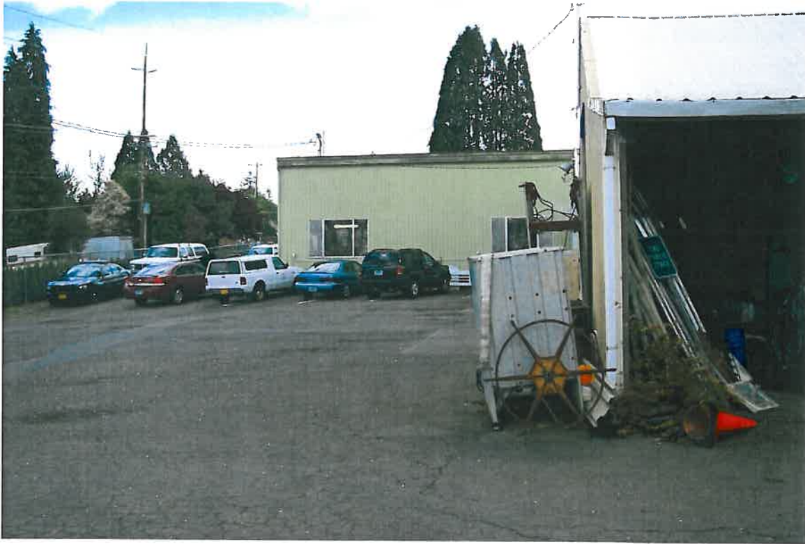
Vehicle Maintenance Shops – Looking North
