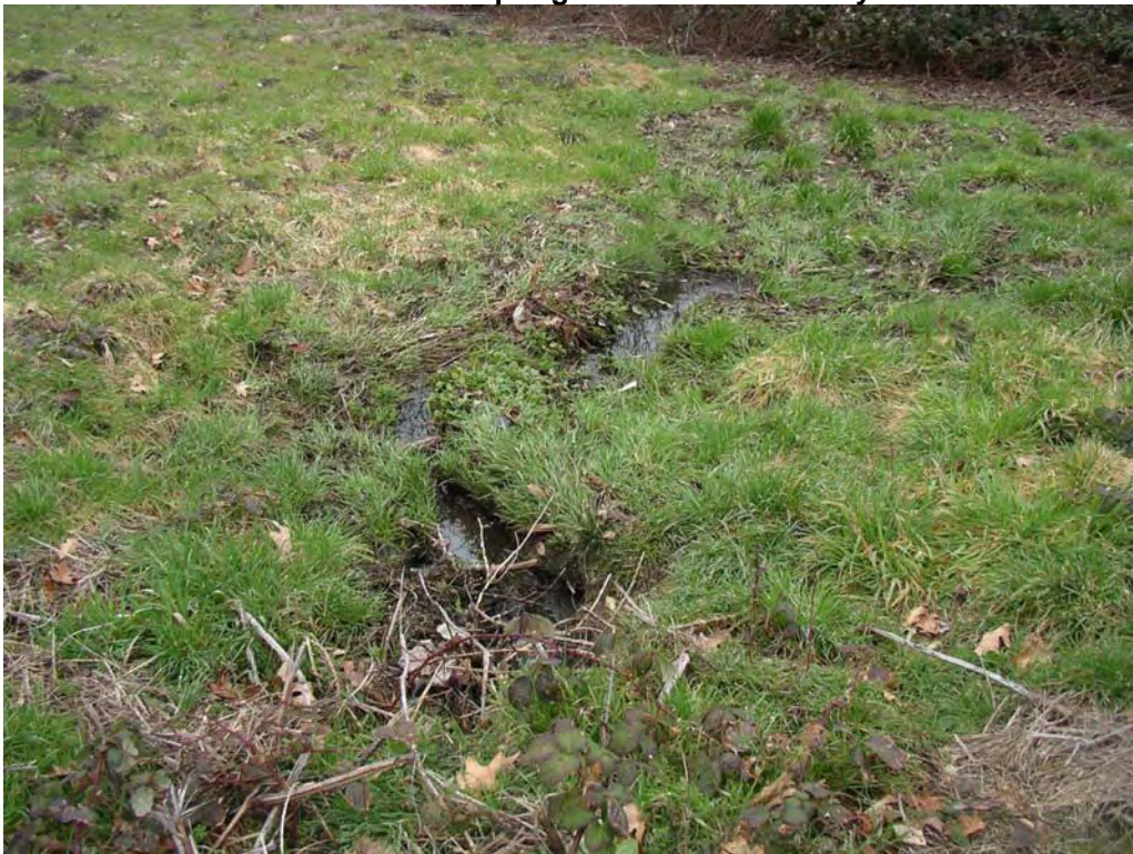
Photo W2 - Hidden Springs Stormwater Conveyance
