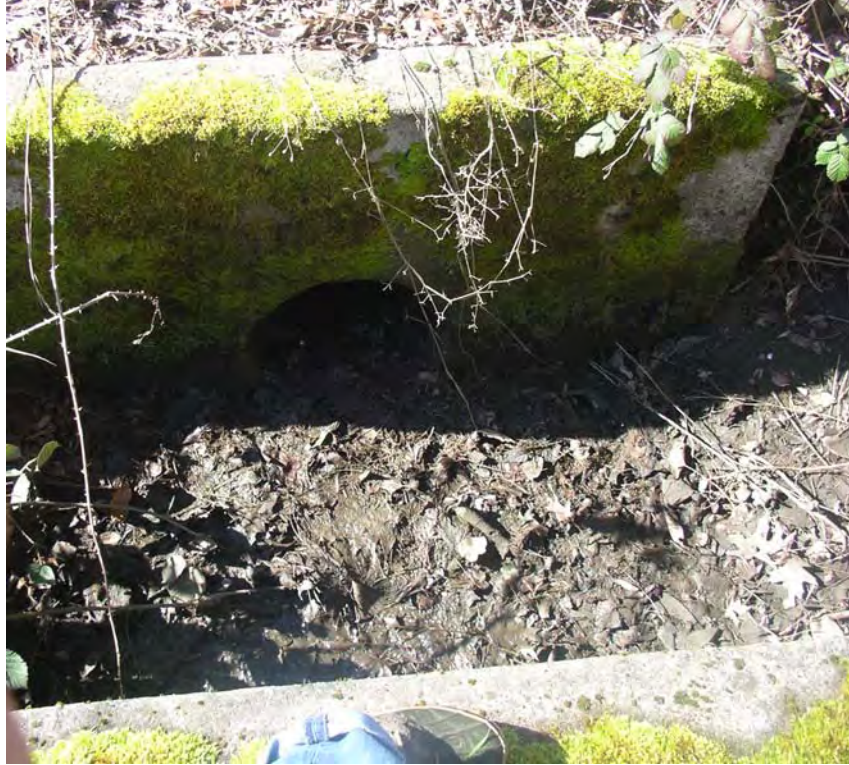
Photo W3 Culvert Under Rosemont Rd Feeds Stormwater Ditch Water 3
