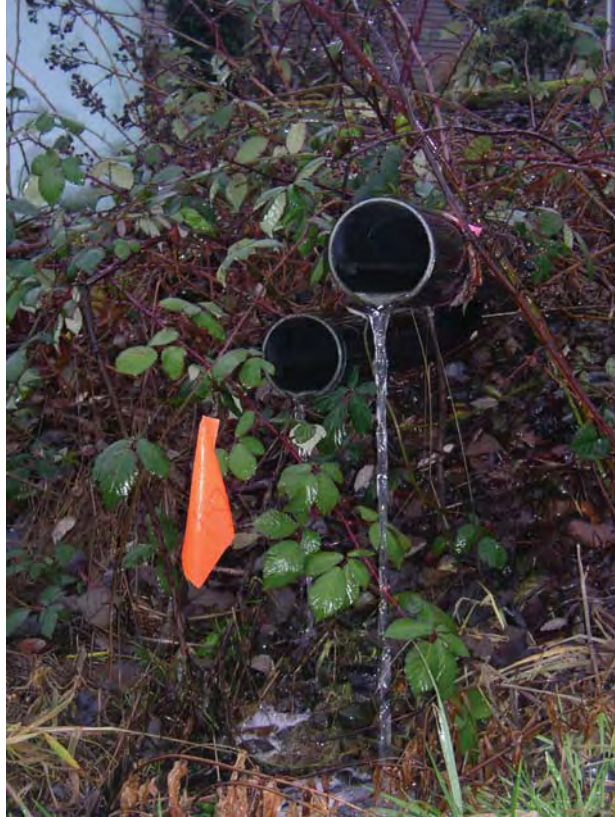
Photo D3 - Source of Hydrology for D1 Plots - Storm Water Outfall Pipes
