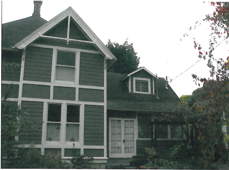
West-facing view of east side of house, area on right will undergo the opening of the enclosed porch, replacement of the dormer with a larger dormer, and expansion of the second story's livable area by raising the east wall of the main body of the house.
