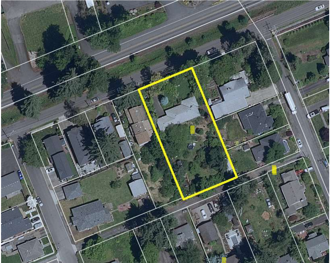
Aerial Photograph of Existing Conditions
