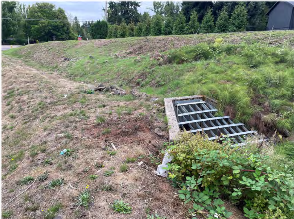
Photo Point 3. Facing east, showing storm drain inlet (September 2023).
