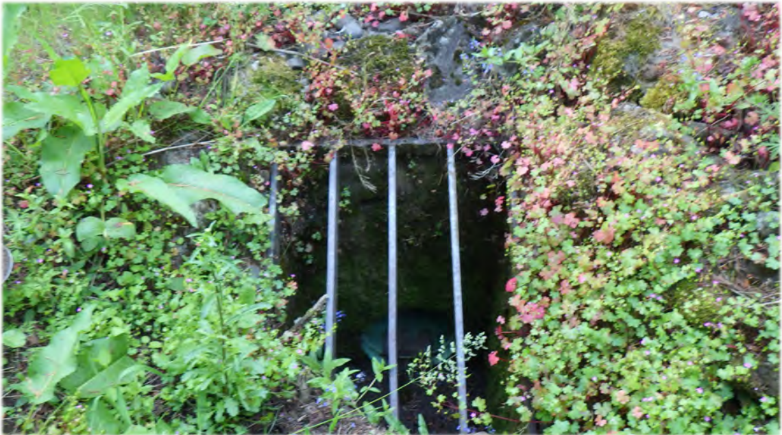
Photo Point 4. From the end of the tributary to Maddax Creek facing southeast toward storm drain.
