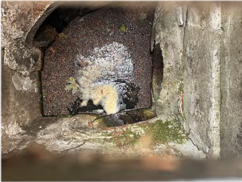
Showing catch basin at Wilderness Park, origin of the tributary – photo provided by applicant 6/4/2026
