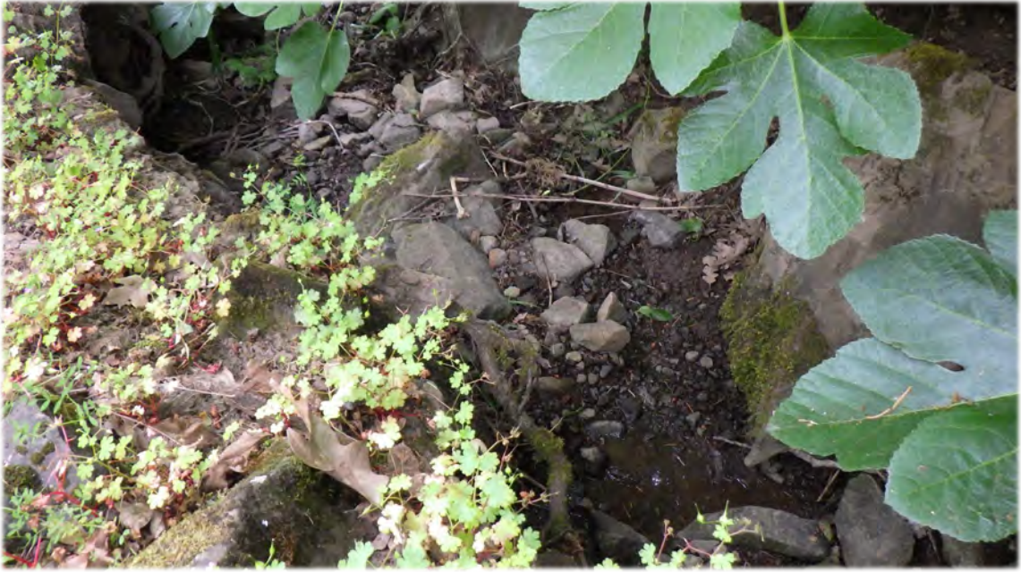
Photo Point 5. Showing significant erosion along steep channel section.
