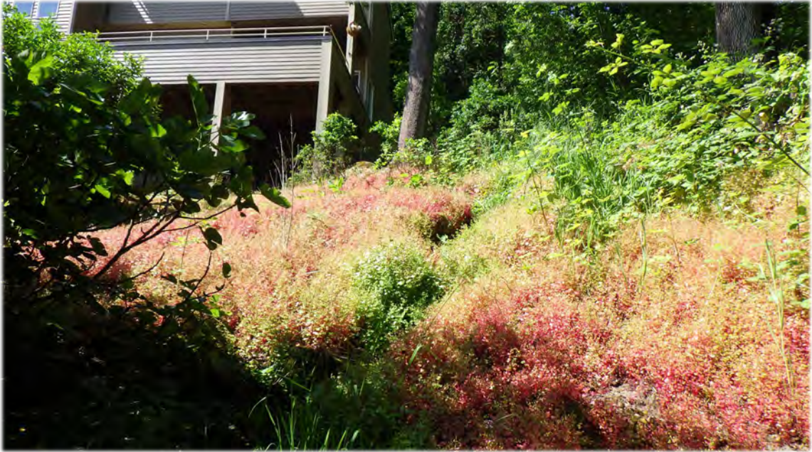
Photo Point 5. Showing steep, eroded northeast drainage section
