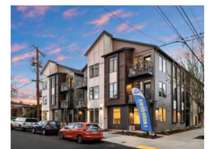
SE 11th & Tenino Apartments Low-Rise Apartments
