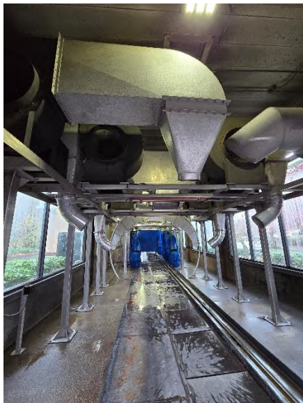
End of Tunnel at Tualatin
