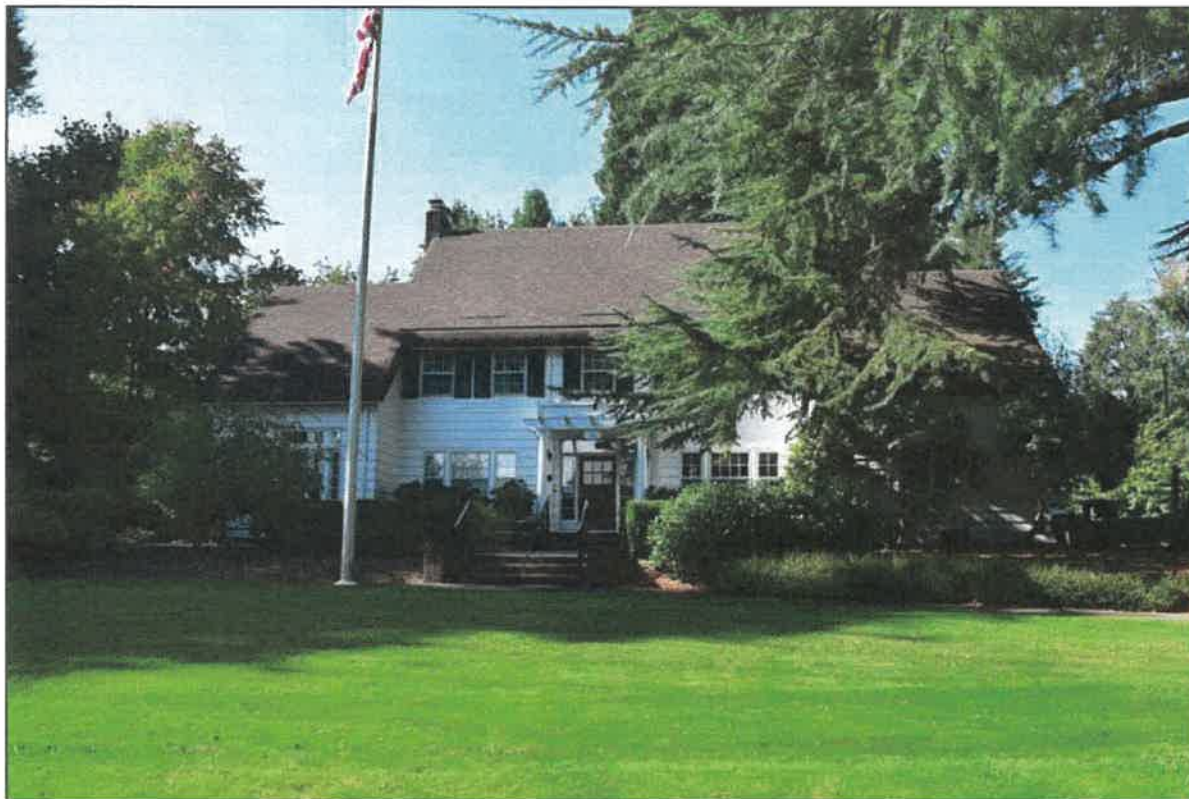
Photo 1 of 15: OR_ClackamasCounty_McLeanHouse_0001 Looking northwest at the front ('east') of the house.
