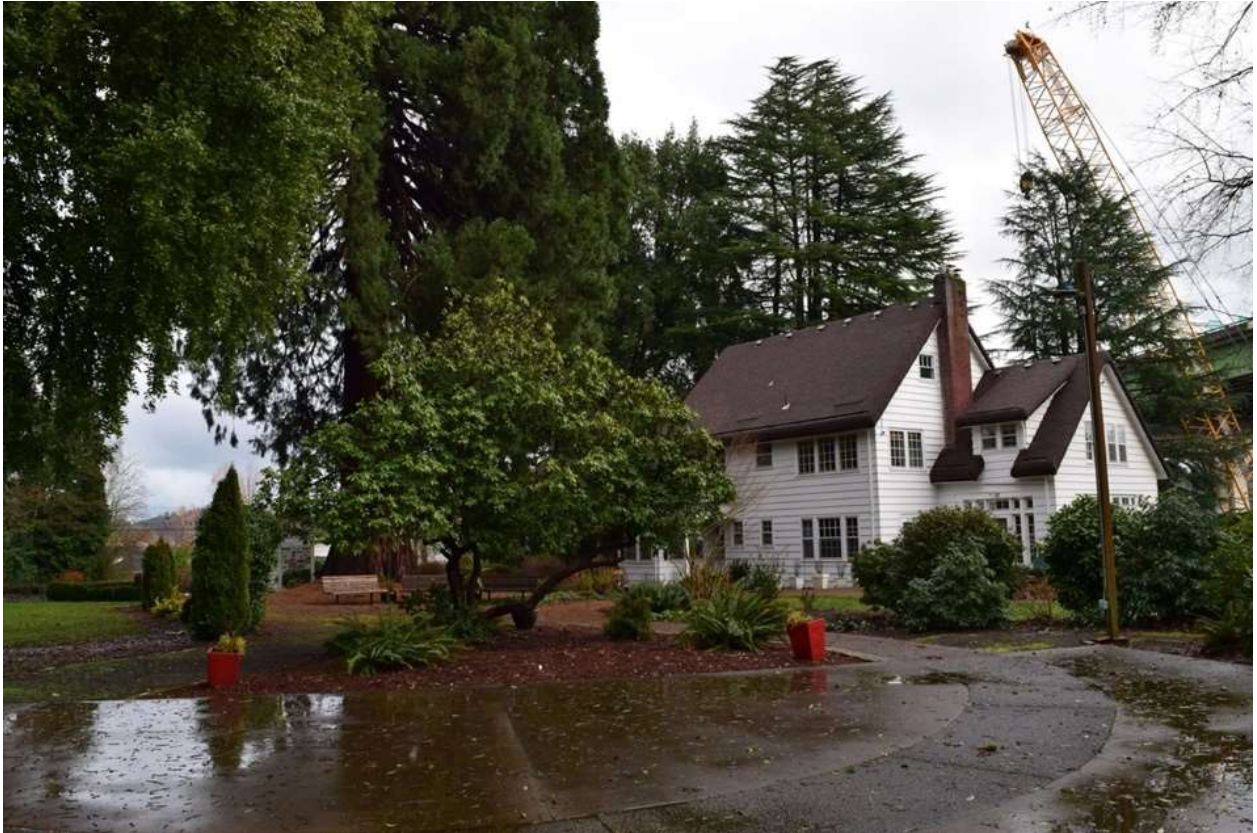
OR_Clackamas_McLeanHouse_0005, Looking east at 'west' and 'south' walls of house and large trees nearby.
