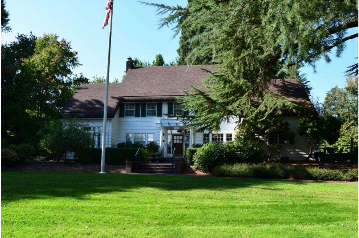
OR_Clackamas_McLeanHouse_0001, Looking northwest at the front ('east') of the house.
