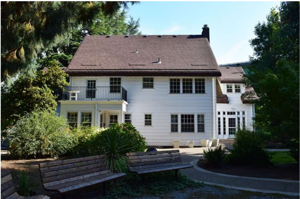
OR_Clackamas_McLeanHouse_0004, Looking southeast at rear façade.
