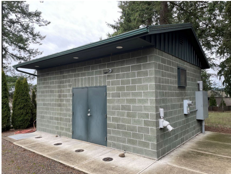
Photo 1-9 | Bland Pump Station
