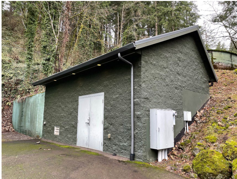
Photo 1-7 | View Drive Pump Station
