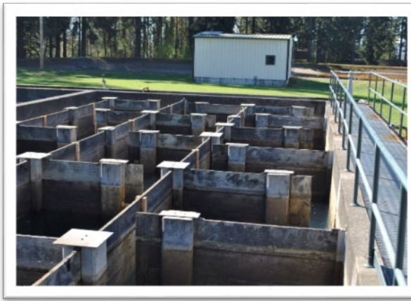
Figure 6-7. Hydraulic Flocculators
