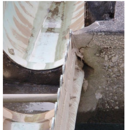
Figure 4-6. Launder Trough Anchorage
