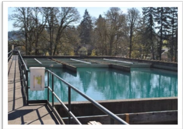
Figure 6-8. Sedimentation Basin
