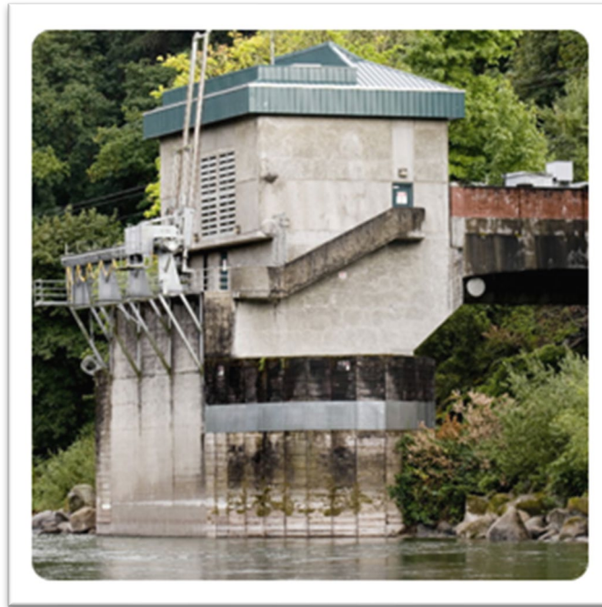
Figure 6-5. SFWB's Intake and RWPS Is in Good Condition and Has a Secondary Power Supply
