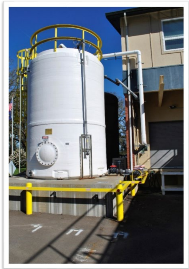
Figure 6-16. Hypochlorite Tanks
