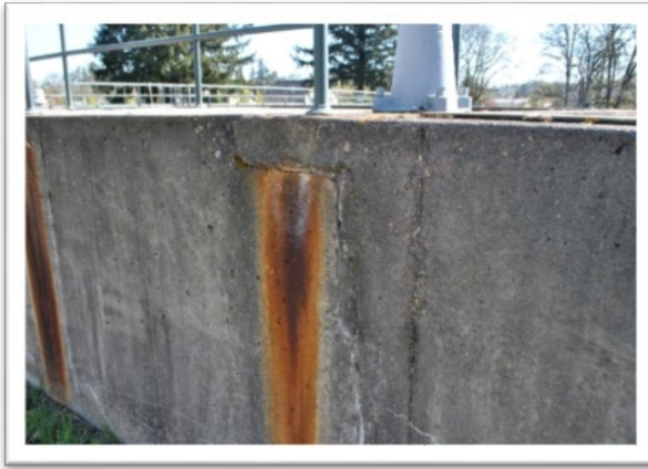
Figure 6-9. Sedimentation Basins Concrete
