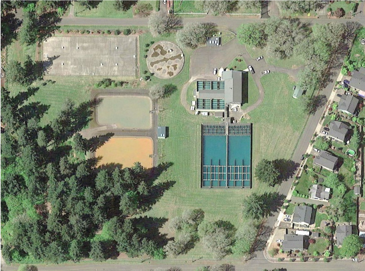
Figure 2-1. SFWB WTP Aerial Photograph
