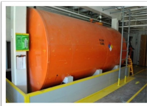
Figure 6-13. Alum Tank
