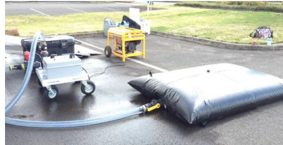
Figure 6-20. Photos of Distribution System Manifolds
