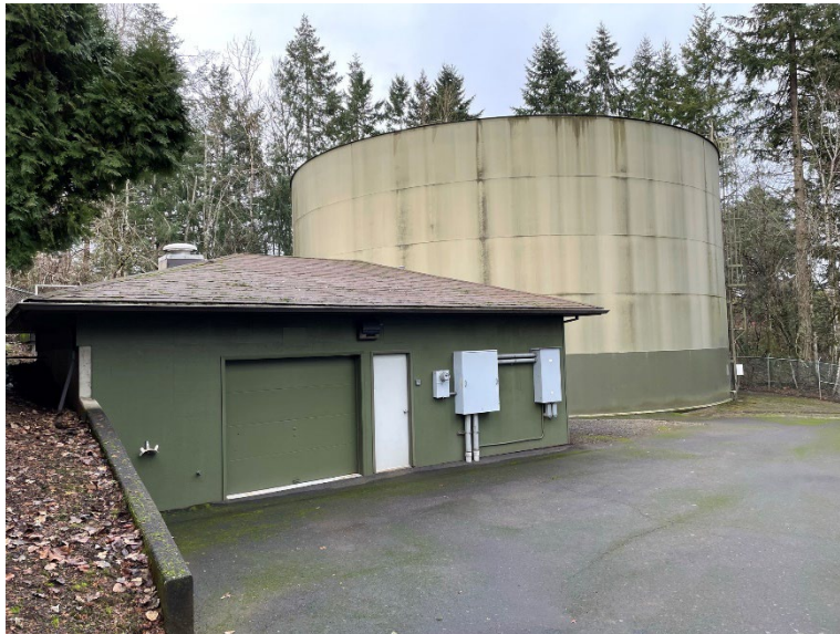
Photo 1-3 | Horton Pump Station
