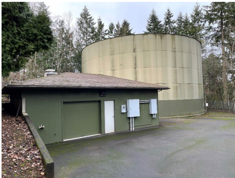
Photo 1-3 | Horton Pump Station
