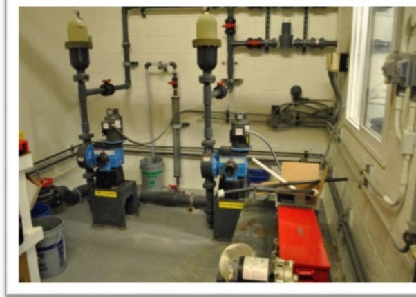
Figure 6-14. Hypochlorite Feed System
