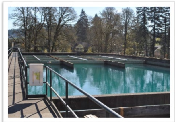
Figure 6-8. Sedimentation Basin
