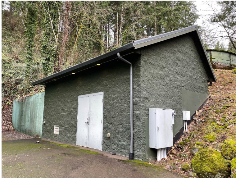
Photo 1-7 | View Drive Pump Station
