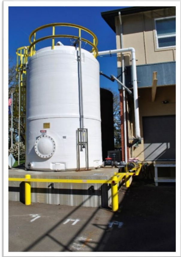
Figure 6-16. Hypochlorite Tanks
