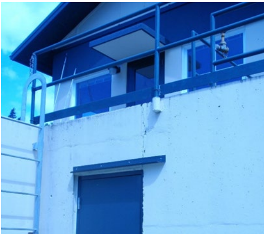
Figure 4-1. Filters Exterior South Wall
