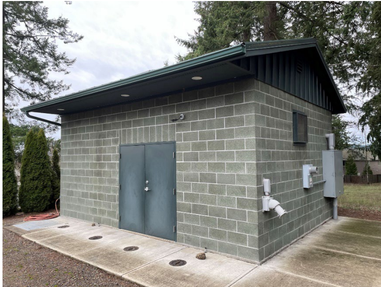
Photo 1-9 | Bland Pump Station
