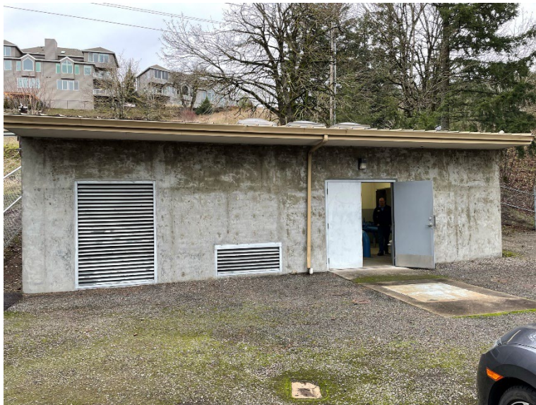
Photo 1-5 | Willamette Pump Station
