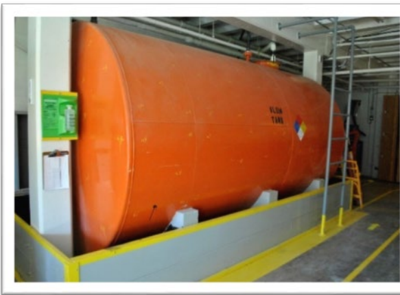
Figure 6-13. Alum Tank
