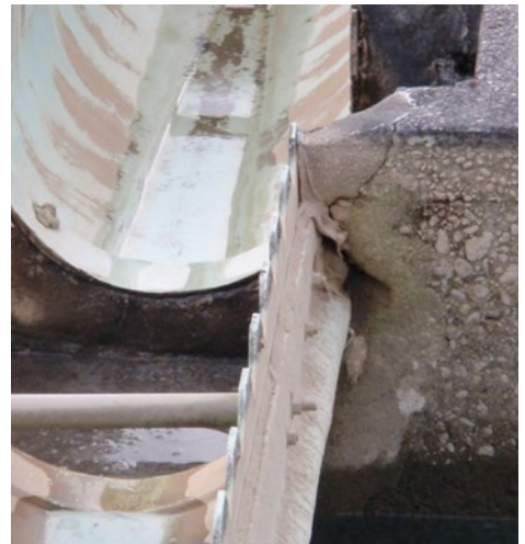
Figure 4-6. Launder Trough Anchorage
