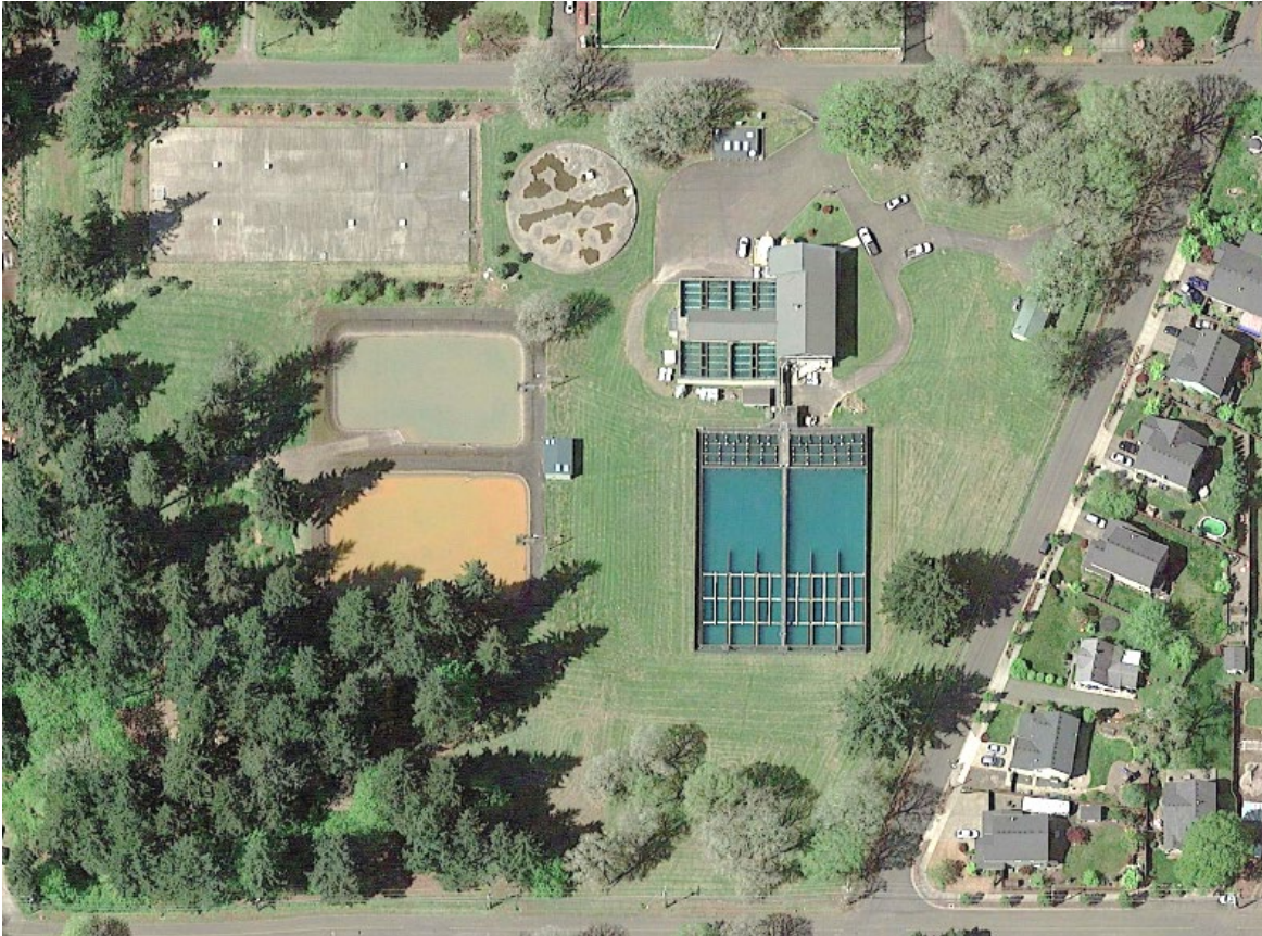
Figure 2-1. SFWB WTP Aerial Photograph
