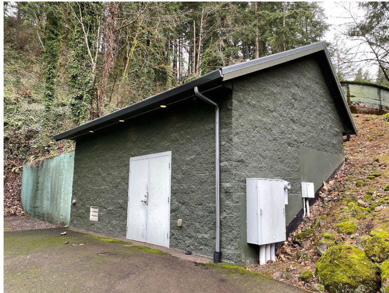
Photo 1-7 | View Drive Pump Station
