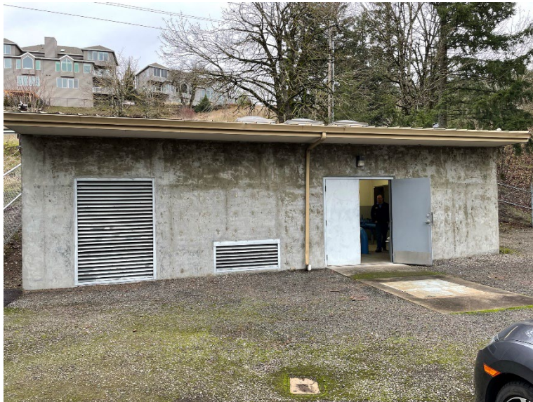
Photo 1-5 | Willamette Pump Station
