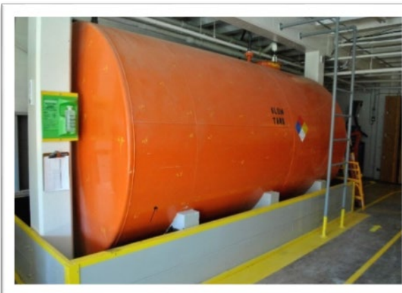
Figure 6-13. Alum Tank
