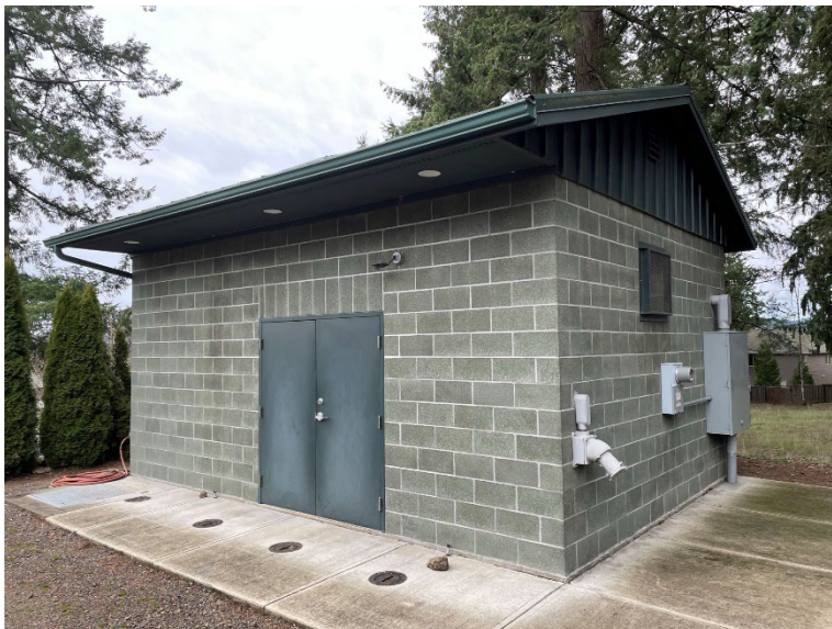
Photo 1-9 | Bland Pump Station
