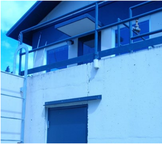
Figure 4-1. Filters Exterior South Wall
