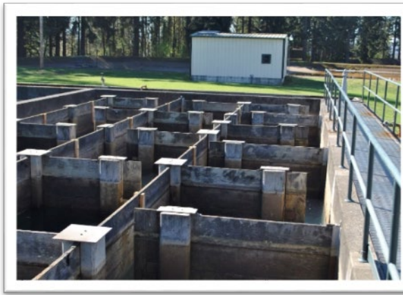
Figure 6-7. Hydraulic Flocculators
