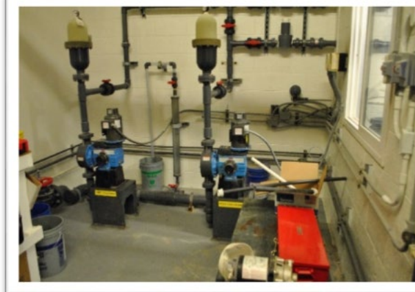
Figure 6-14. Hypochlorite Feed System
