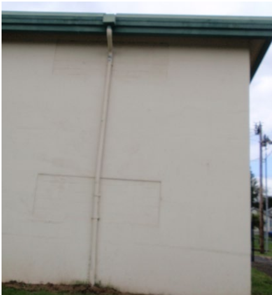
Figure 4-7. DSPS Exterior Wall Corner
