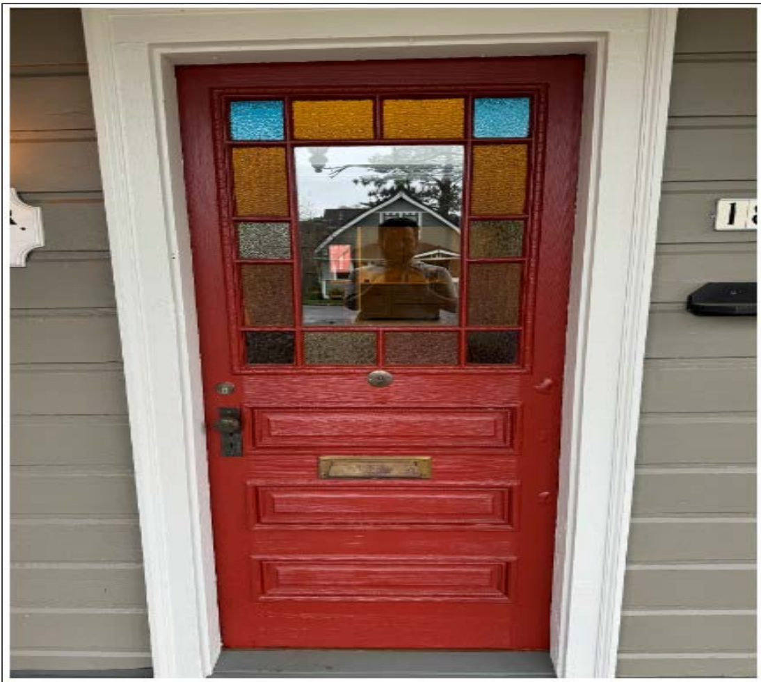
Existing Front Door (Facing 5 th Ave)
