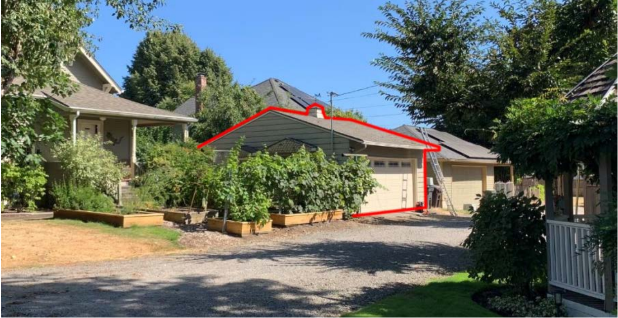
Rear Facing façade of the home and garage structure viewed from 15 th St. in 2023. Note the neighboring garage structure has a system very similar to that which the applicant is proposing for theirs.
