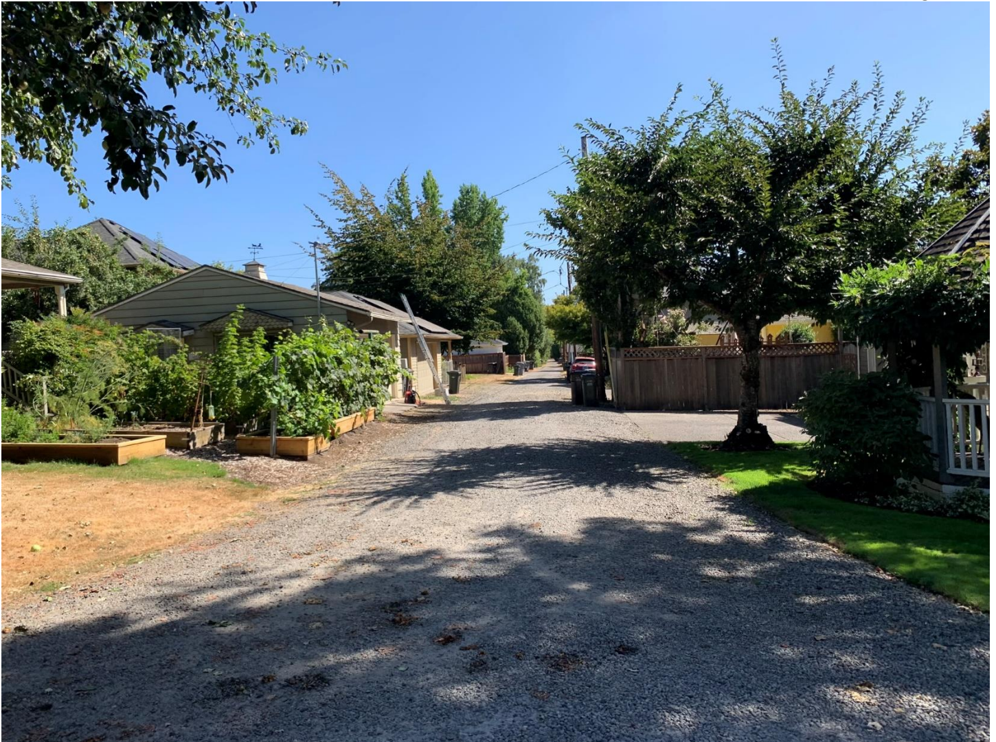
Figure 5: View of the rear of the garage from the Alley off of 15th Street
