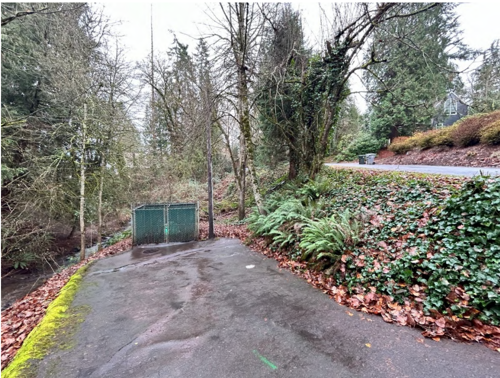
Existing driveway and pump station below Calaroga Drive. New pump station to be constructed in the area to the right of the fenced enclosure.
