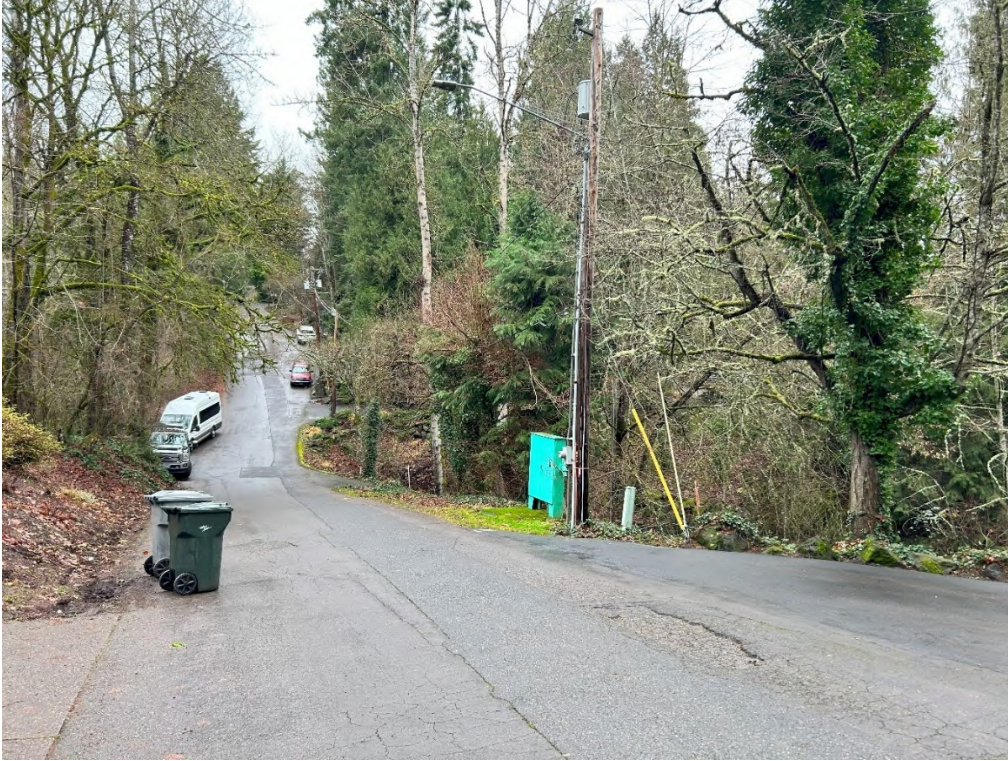
View of the existing pump station and Calaroga Drive, looking west. Proposed project to be located in the vicinity of the existing control box (center of image).
