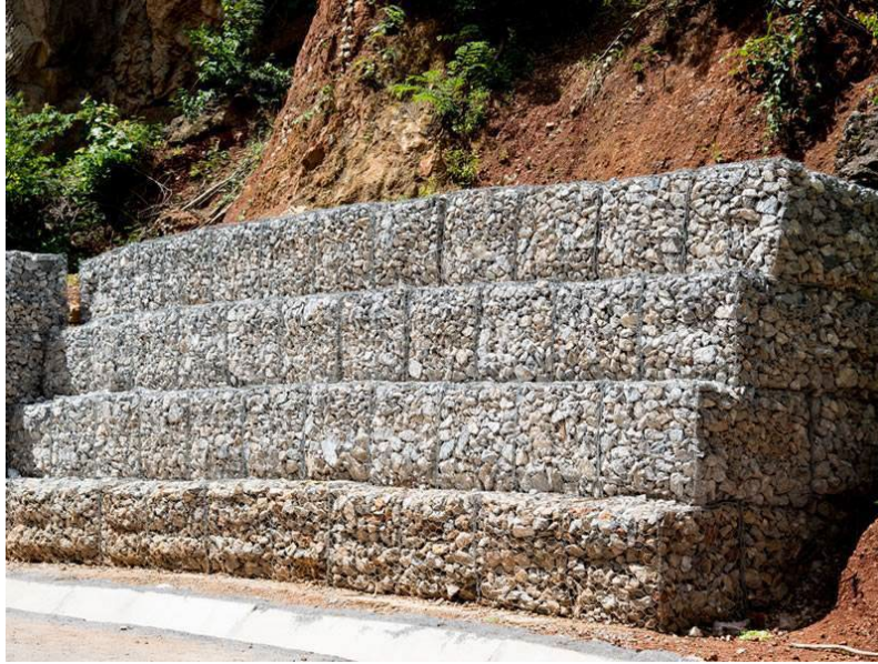
Examples of Rock Gabion Walls
