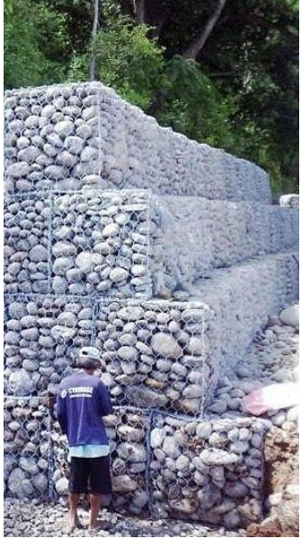
Examples of Rock Gabion Walls
