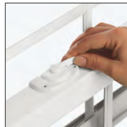
Press the tilt release button and slide the lock lever over the button.
