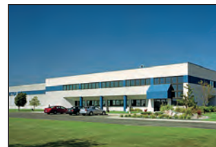
Our facilities eliminate 95% or more of VOCs (Volatile Organic Compounds).
