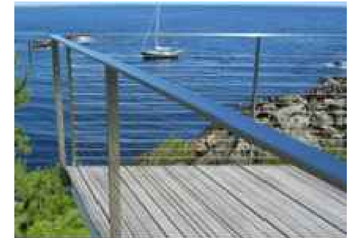
02 CONCEPT PHOTO: DECK RAILING - STEEL AND TENSION WIRE
