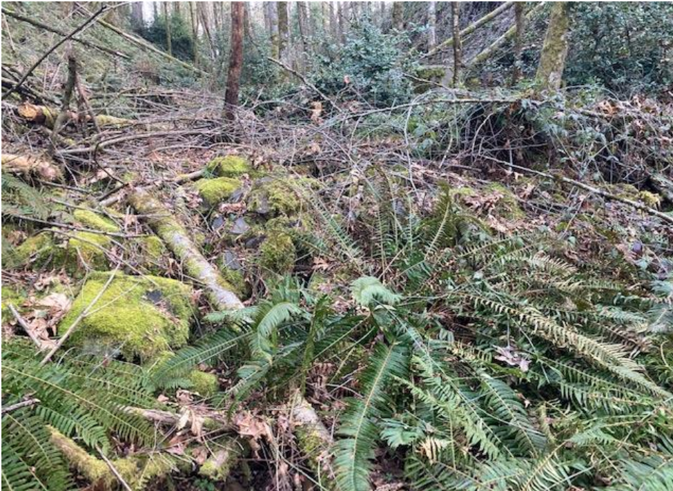
Photo 5 showing rocky (rip-rap) impoundment across Robin Creek drainage above subject property near City's concrete storm drain structures (middle back right) discovered on March 16, 2023
