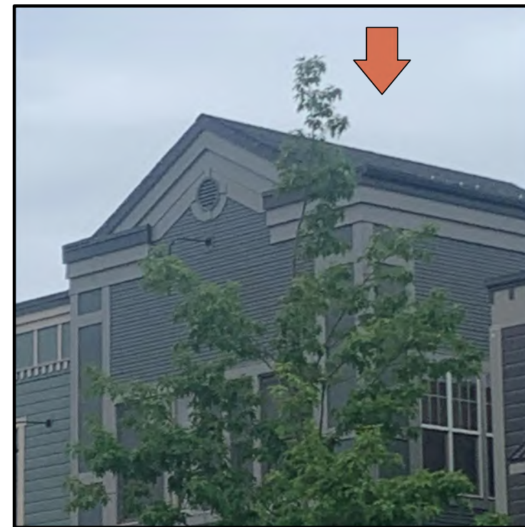
1980 WFD: 3rd FLOOR 1,735 SF ROOF SPACE
