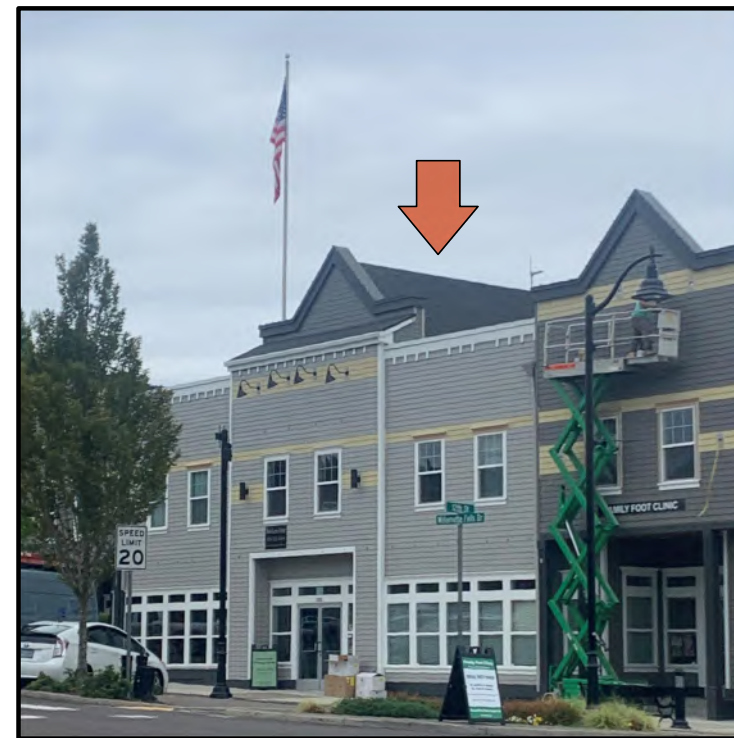
1914 WFD: 3rd FLOOR 330 SF ROOF SPACE
