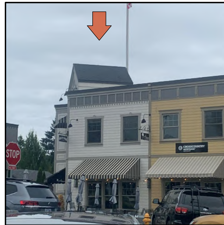
1914 WFD: 3rd FLOOR 200 SF ROOF SPACE
