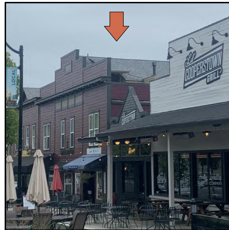
1849 WFD: 3rd FLOOR 1,710 SF ROOF SPACE
