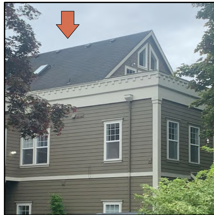
1672 WFD: 3rd FLOOR VIEW FROM REAR
