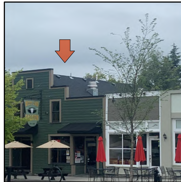
1880 WFD: 3rd FLOOR 530 SF ROOF SPACE
