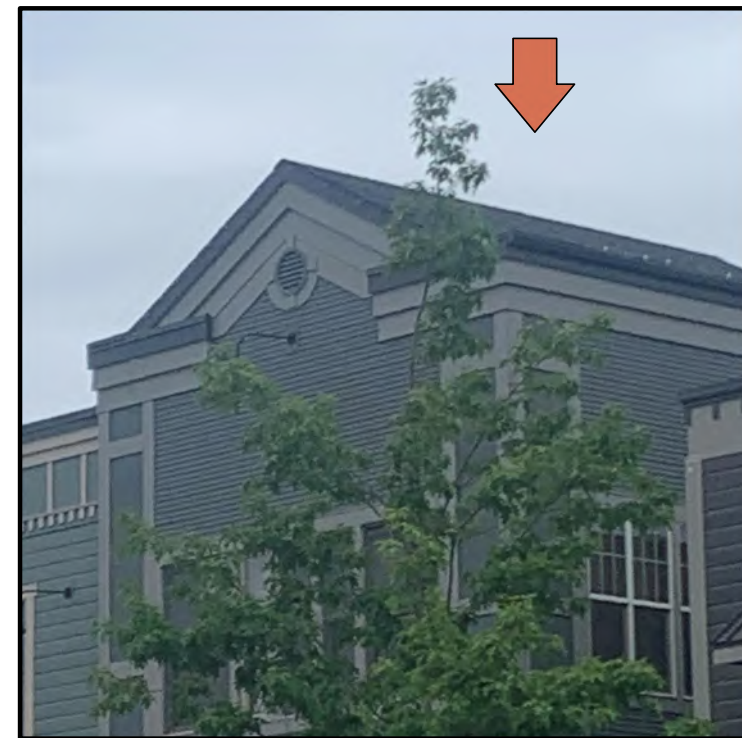
1980 WFD: 3rd FLOOR 1,735 SF ROOF SPACE
