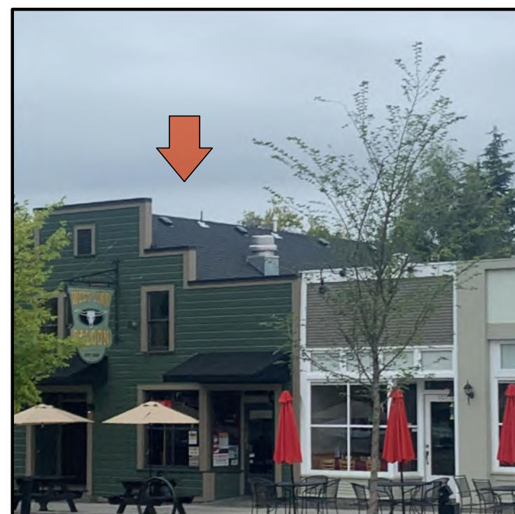
1880 WFD: 3rd FLOOR 530 SF ROOF SPACE
