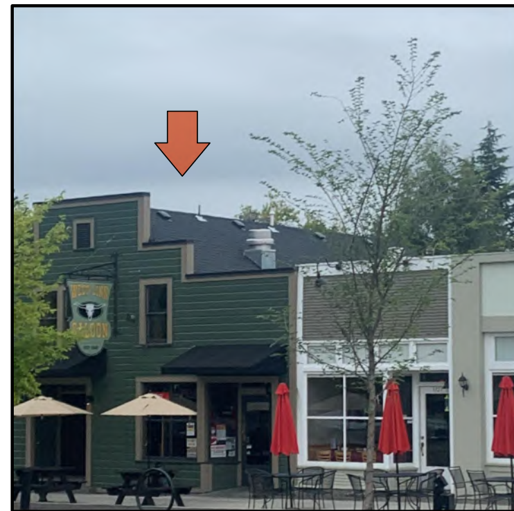
1880 WFD: 3rd FLOOR 530 SF ROOF SPACE
