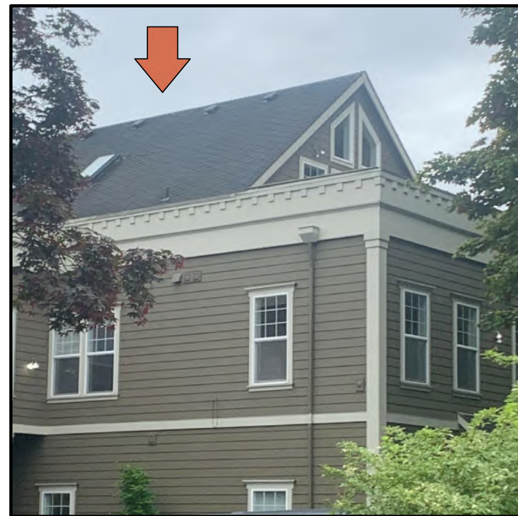
1672 WFD: 3rd FLOOR VIEW FROM REAR
