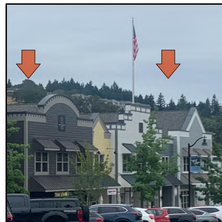
1980 WFD: 3rd FLOOR 1,940 SF ROOF SPACE
