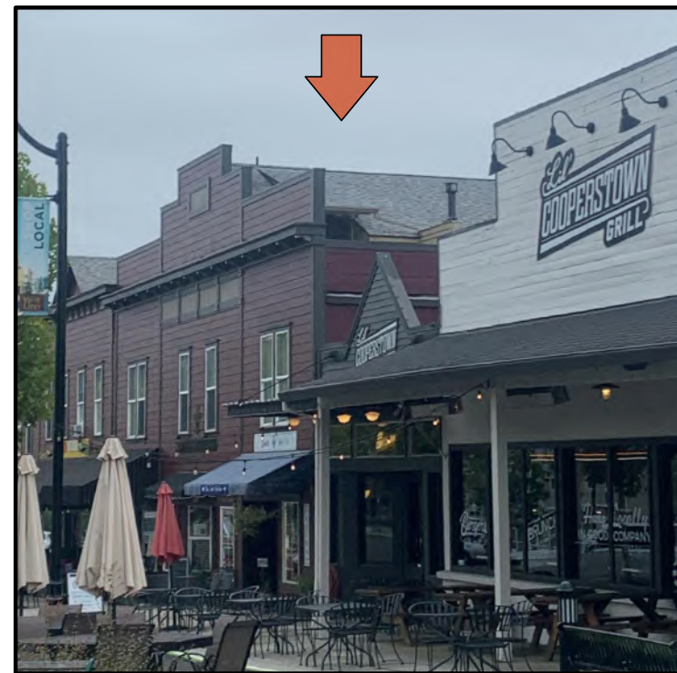
1849 WFD: 3rd FLOOR 1,710 SF ROOF SPACE
