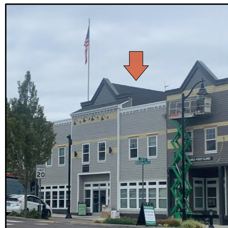
1914 WFD: 3rd FLOOR 330 SF ROOF SPACE
