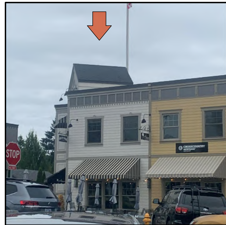
1914 WFD: 3rd FLOOR 200 SF ROOF SPACE
