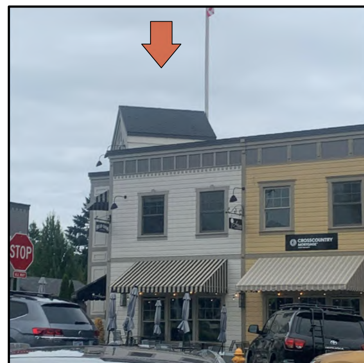
1914 WFD: 3rd FLOOR 200 SF ROOF SPACE
