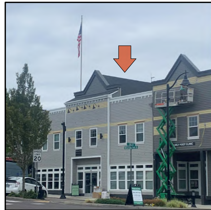
1914 WFD: 3rd FLOOR 330 SF ROOF SPACE
