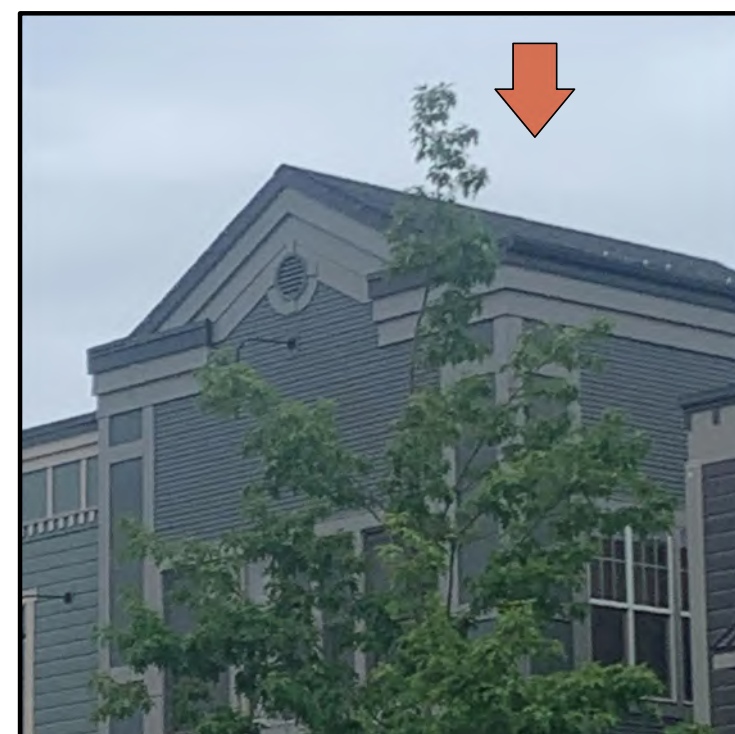
1980 WFD: 3rd FLOOR 1,735 SF ROOF SPACE
