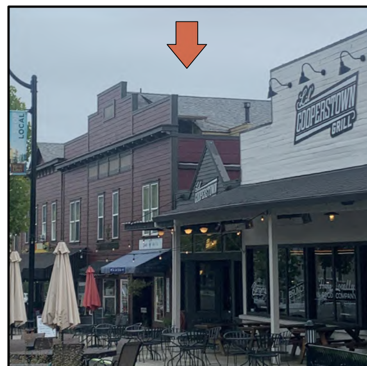
1849 WFD: 3rd FLOOR 1,710 SF ROOF SPACE
