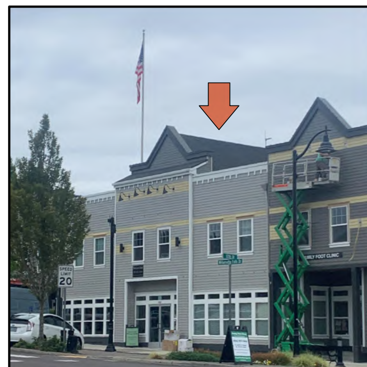
1914 WFD: 3rd FLOOR 330 SF ROOF SPACE
