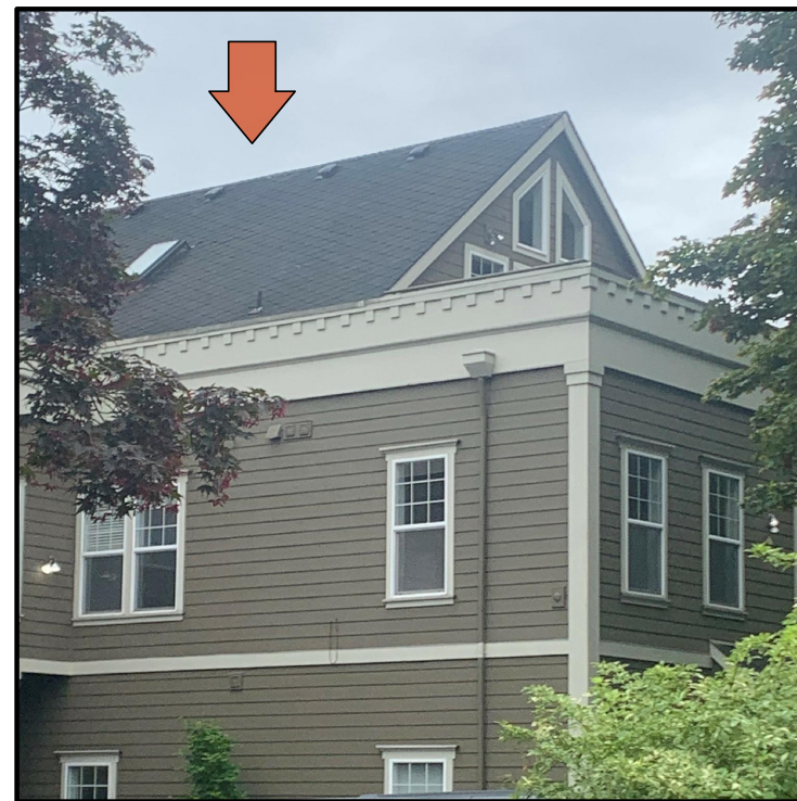
1672 WFD: 3rd FLOOR VIEW FROM REAR
