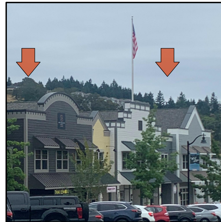
1980 WFD: 3rd FLOOR 1,940 SF ROOF SPACE
