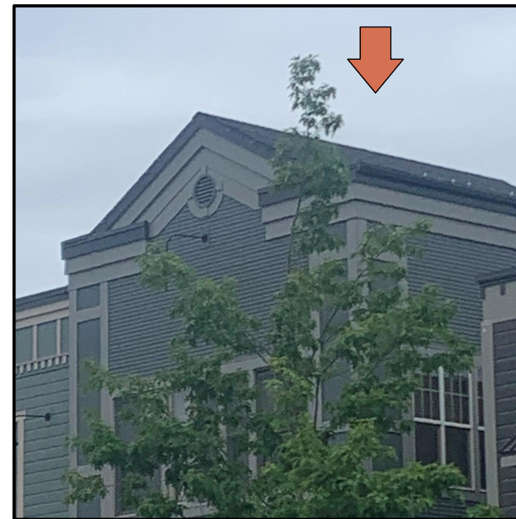
1980 WFD: 3rd FLOOR 1,735 SF ROOF SPACE
