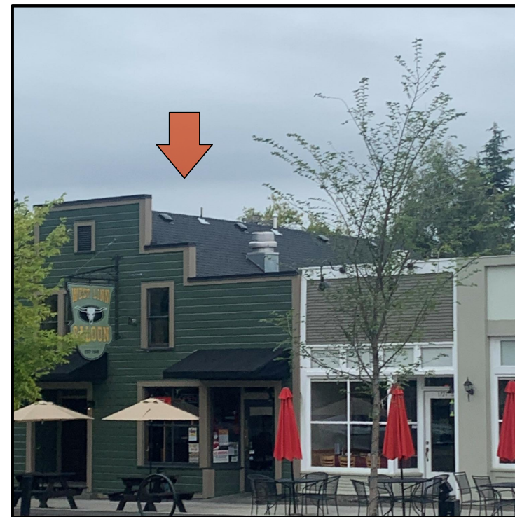
1880 WFD: 3rd FLOOR 530 SF ROOF SPACE
