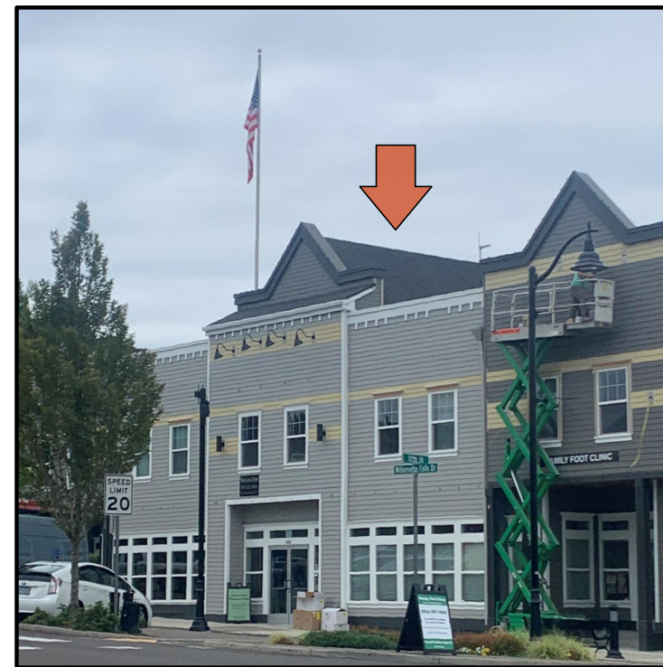
1914 WFD: 3rd FLOOR 330 SF ROOF SPACE
