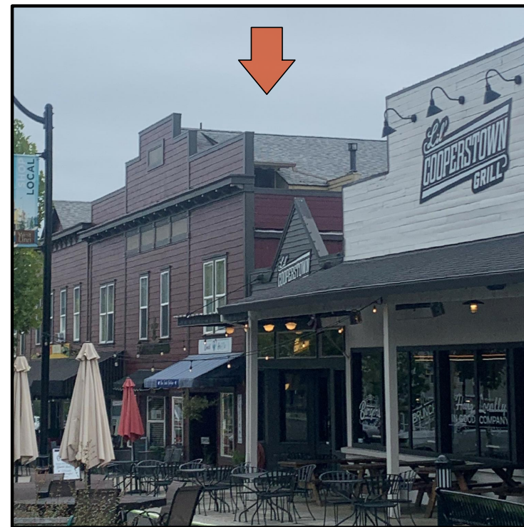
1849 WFD: 3rd FLOOR 1,710 SF ROOF SPACE
