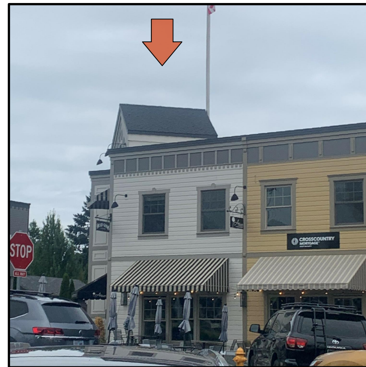
1914 WFD: 3rd FLOOR 200 SF ROOF SPACE
