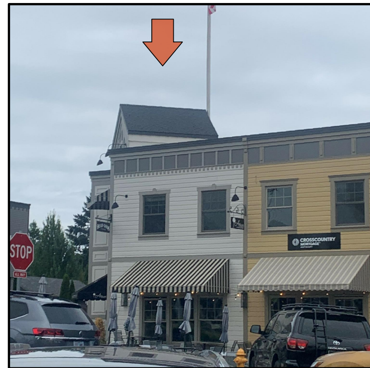
1914 WFD: 3rd FLOOR 200 SF ROOF SPACE
