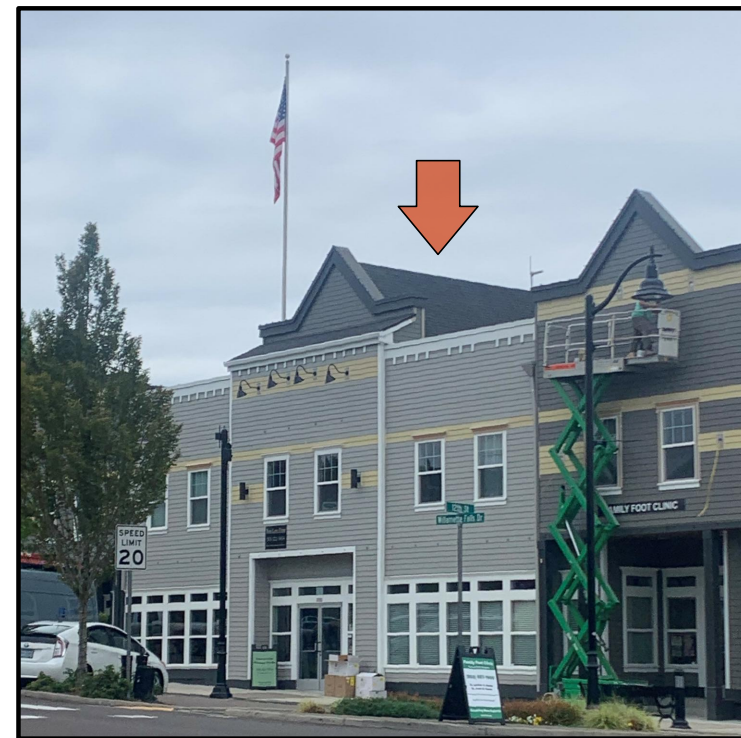
1914 WFD: 3rd FLOOR 330 SF ROOF SPACE
