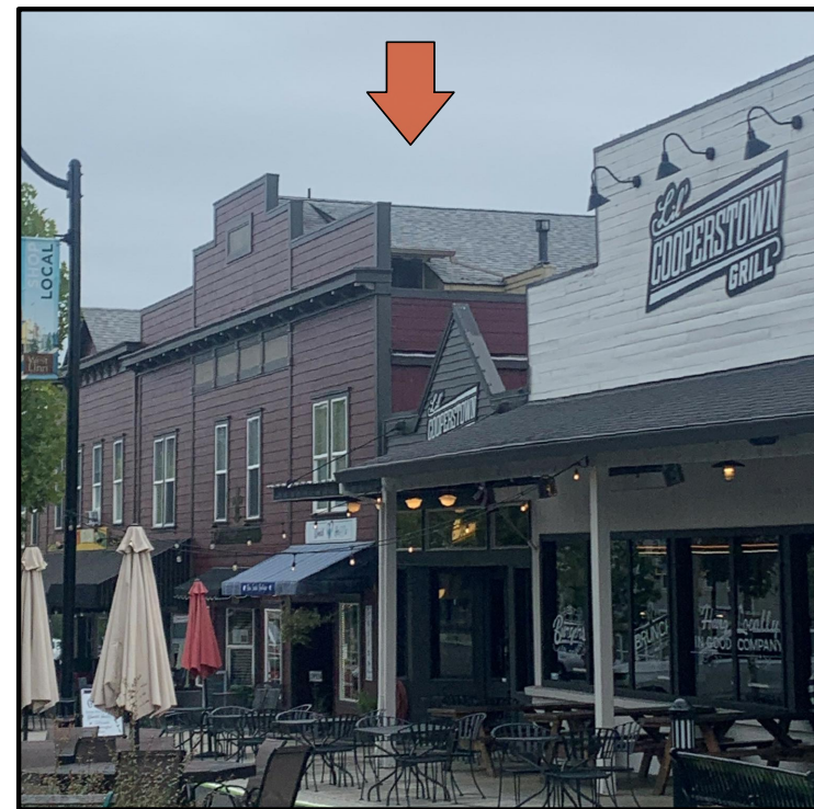
1849 WFD: 3rd FLOOR 1,710 SF ROOF SPACE
