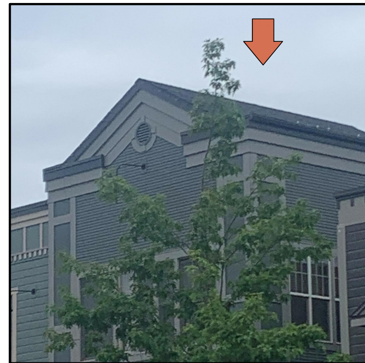
1980 WFD: 3rd FLOOR 1,735 SF ROOF SPACE
