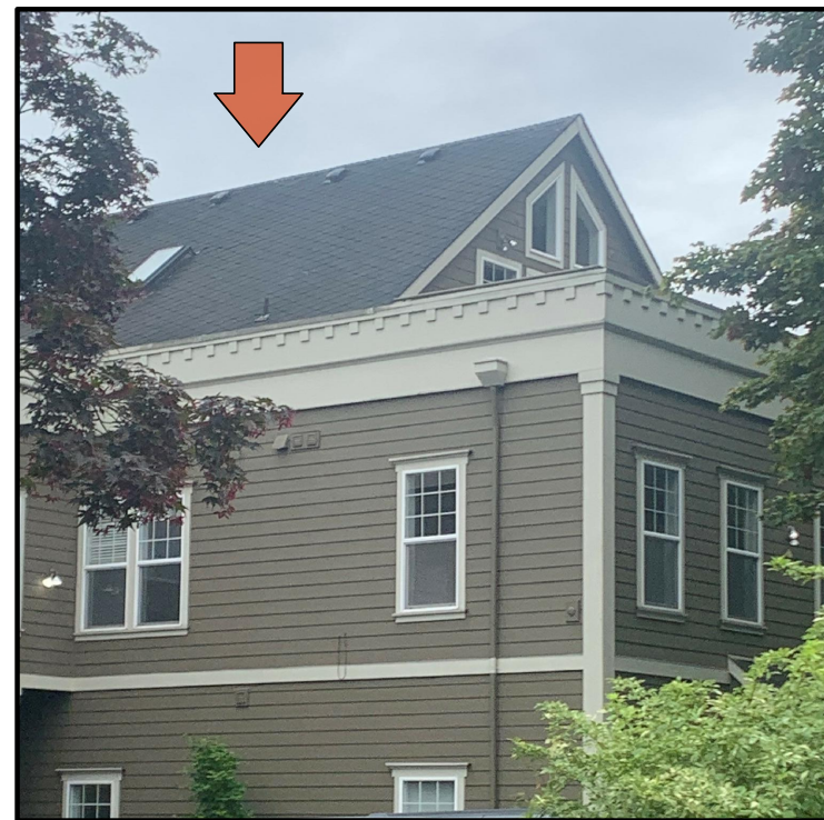
1672 WFD: 3rd FLOOR VIEW FROM REAR
