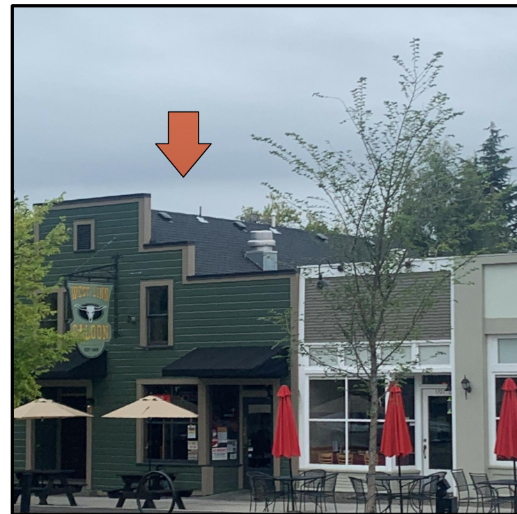
1880 WFD: 3rd FLOOR 530 SF ROOF SPACE
