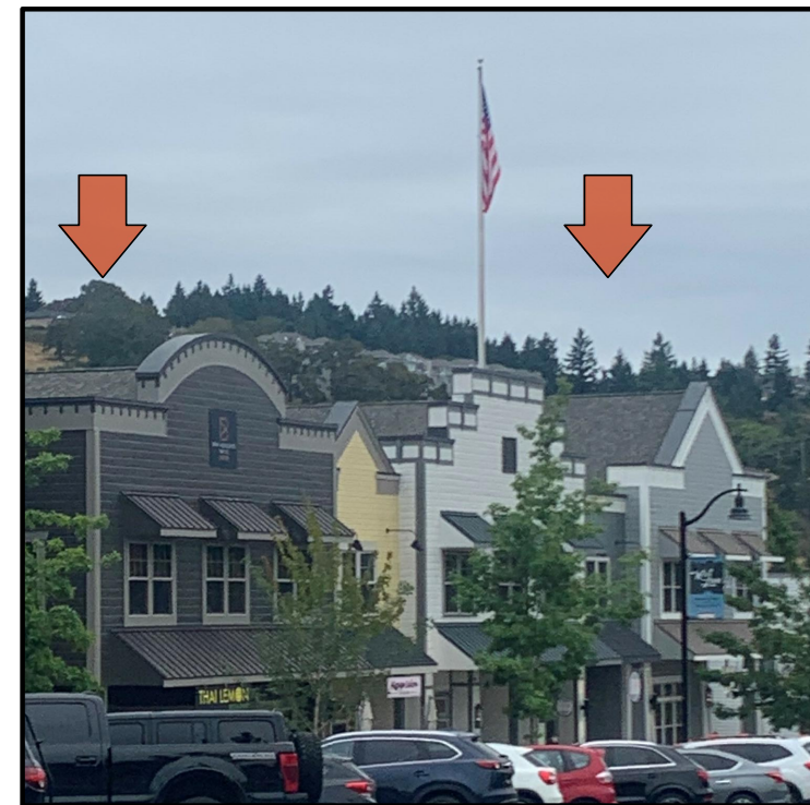
1980 WFD: 3rd FLOOR 1,940 SF ROOF SPACE
