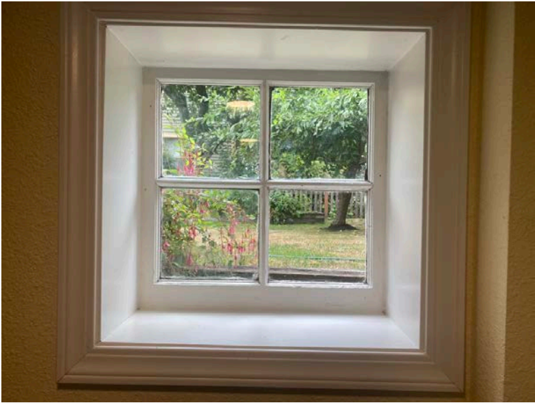
Yard-facing window, interior
