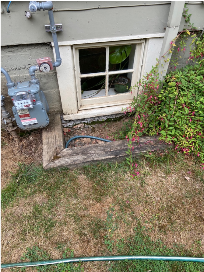
Side yard facing window exterior
