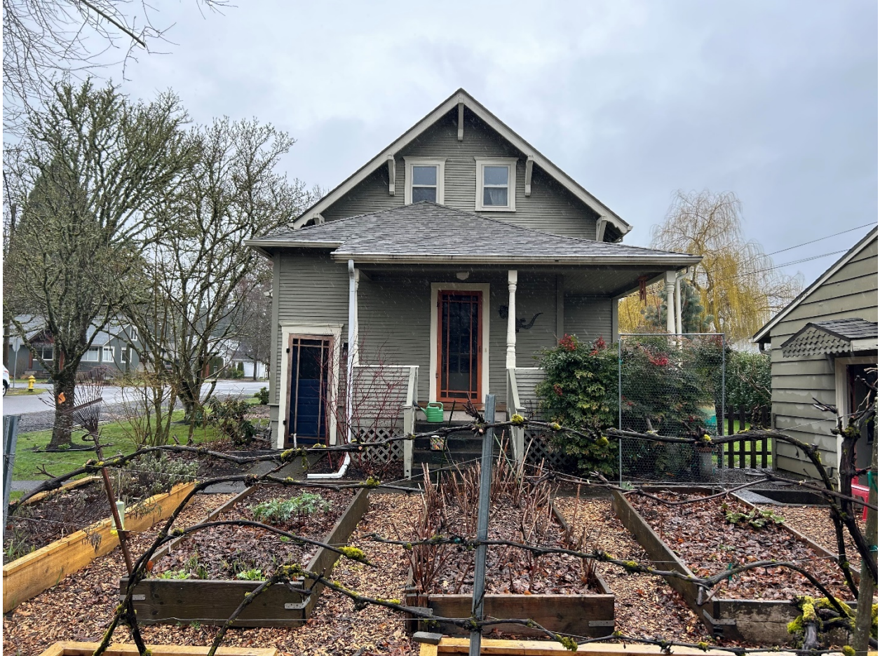
Alley Facing Façade – Door to be replaced in center.
