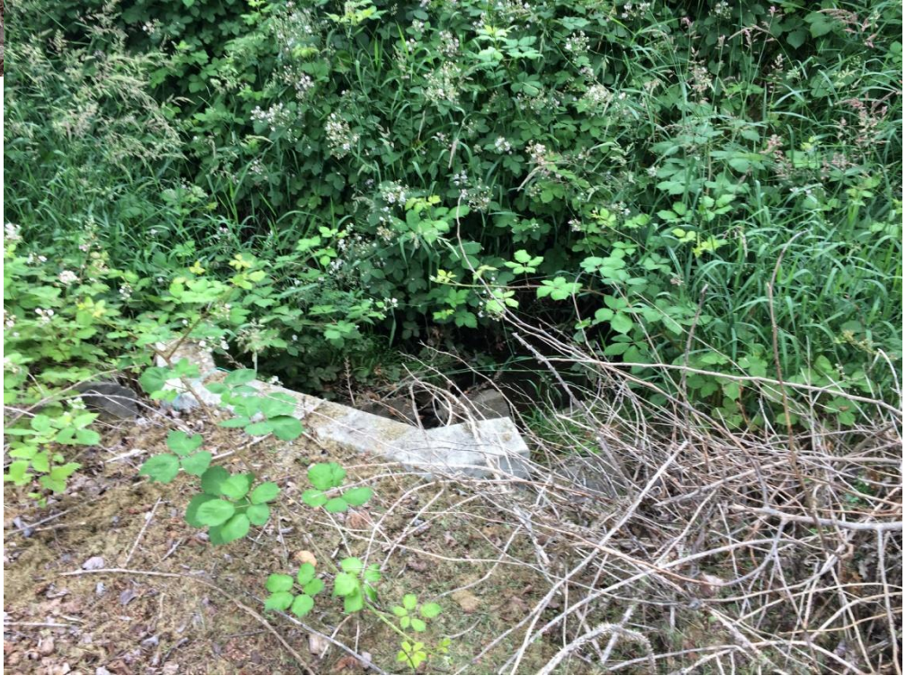
PP1 facing northeast along drainage
