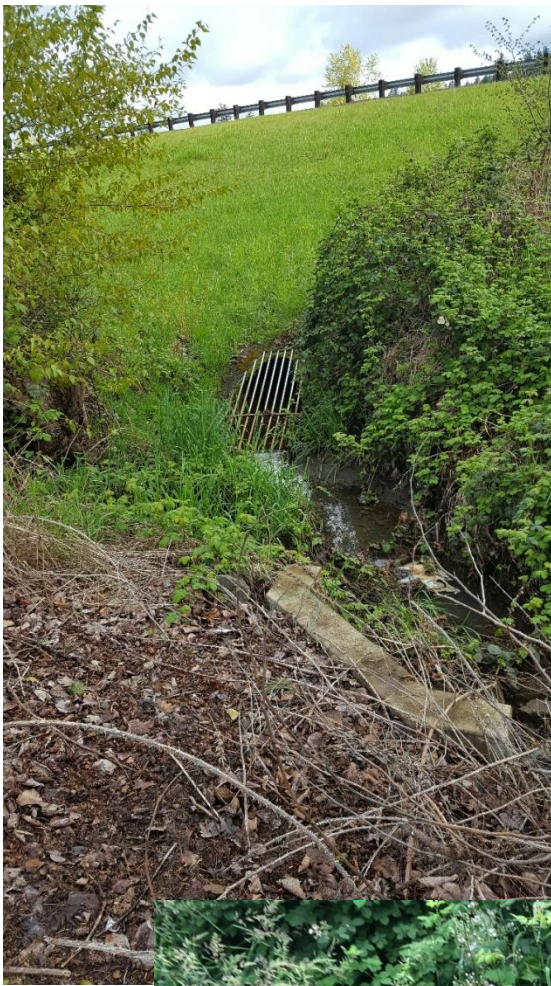
PP1 facing north to culvert under I-205
