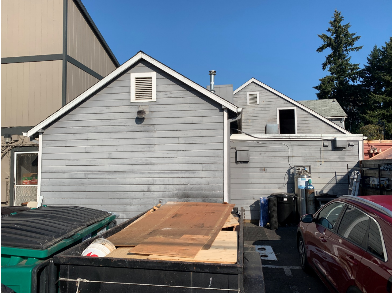
Rear of structure as seen from Knapps Alley.
