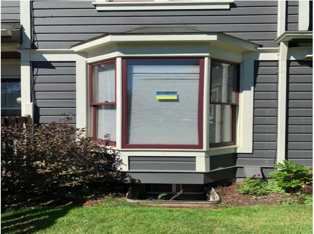
View of the window well where the vinyl window will go
