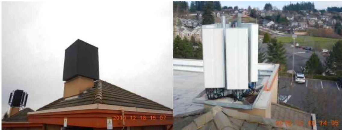
Figure 2: Photographs of existing site
