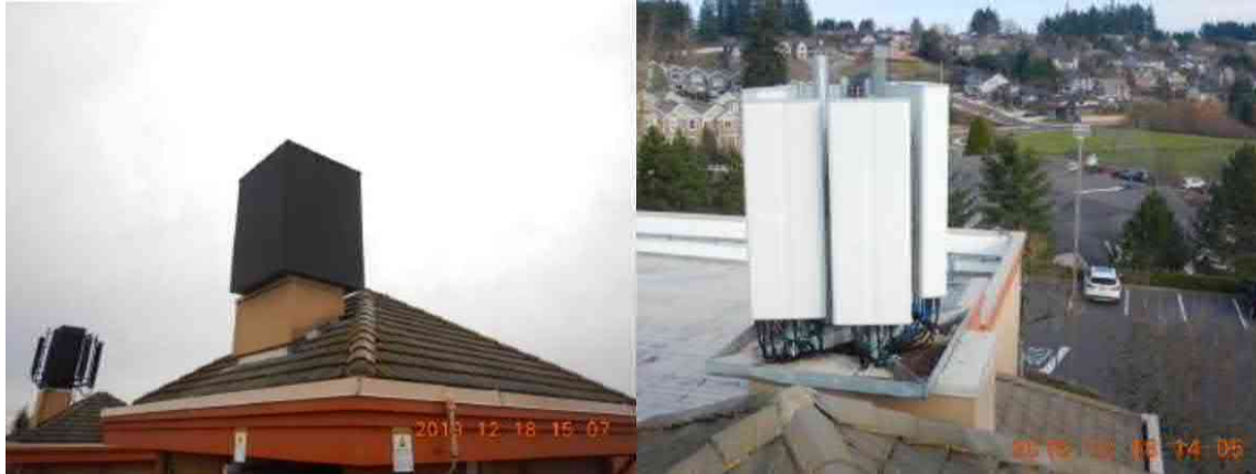
Figure 2: Photographs of existing site
