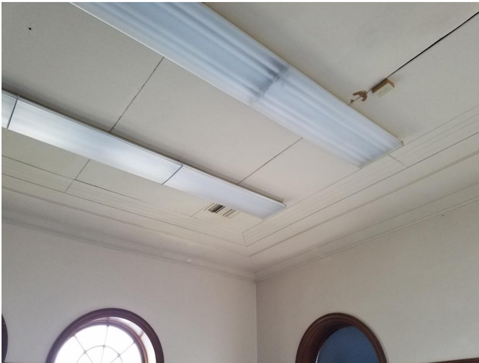
Original Ceiling Detail with existing light fixtures
