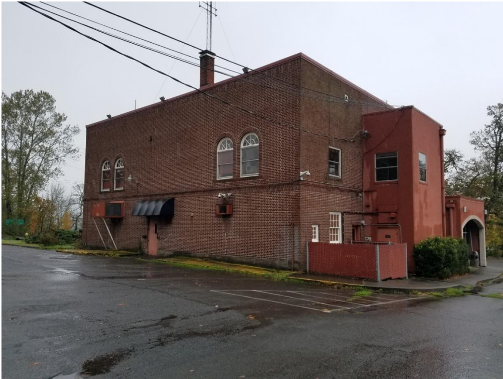
Right and Rear Facades
