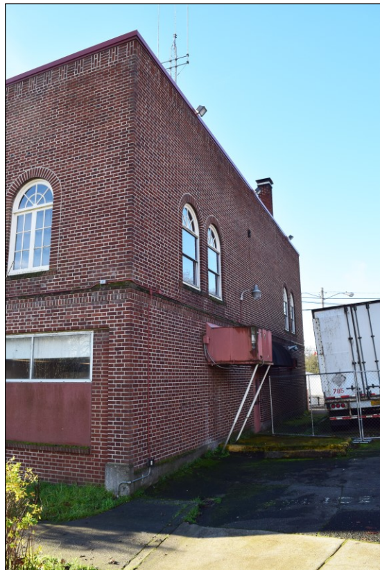
Photo 6 of 13: OR_Clackamas_HistoricCityHall_0006. View of west elevation, looking south.
