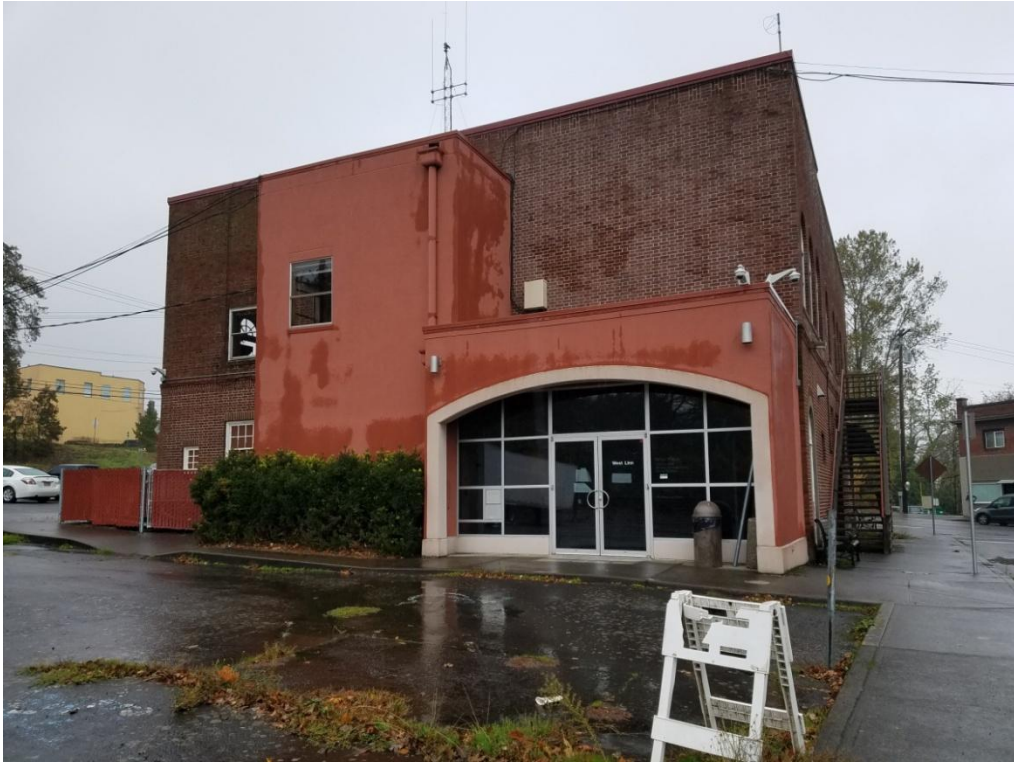
Rear Façade with 1980's addition
