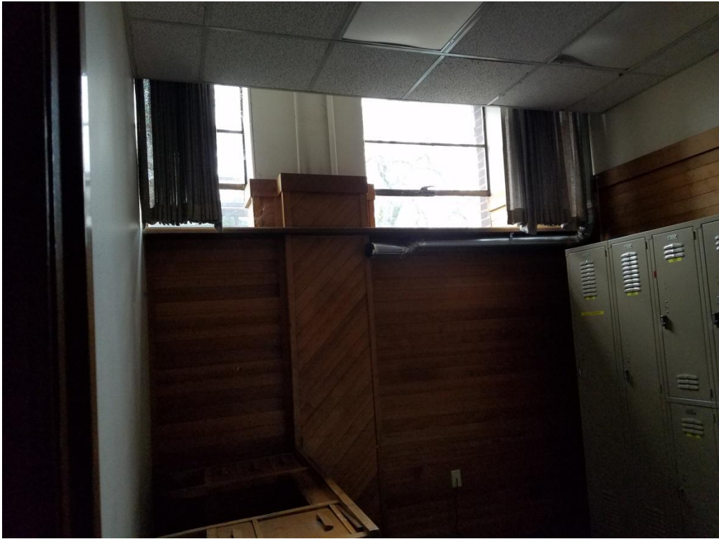
Main Level Offices along Mill St
