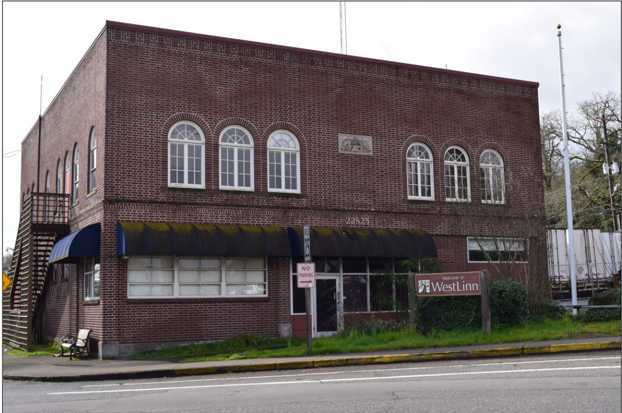
Photo 3 of 13: OR_Clackamas_HistoricCityHall_0003. Looking southwest at the front (north) and east sides.
