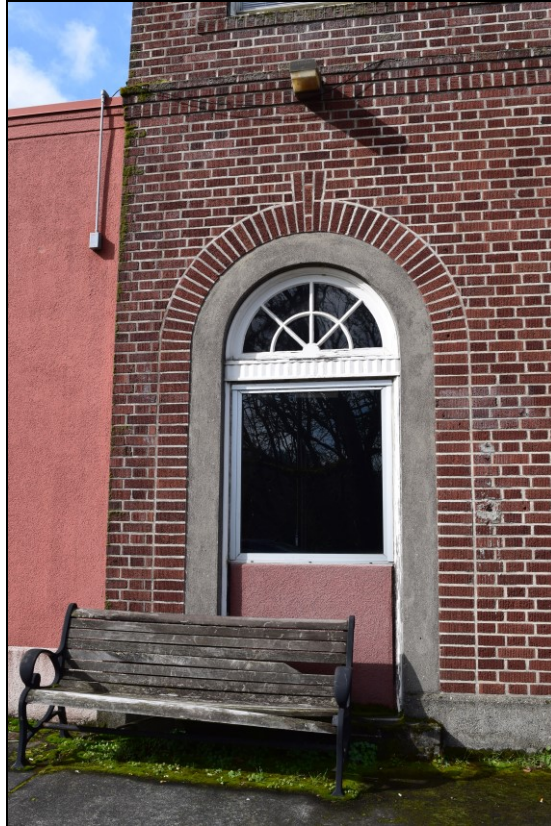
Photo 7 of 13: OR_Clackamas_HistoricCityHall_0007. Looking northwest at the original door opening leading upstairs (now a window) in the east wall.
